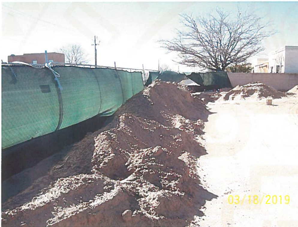
Dirt pile too high above and against silt fence.
