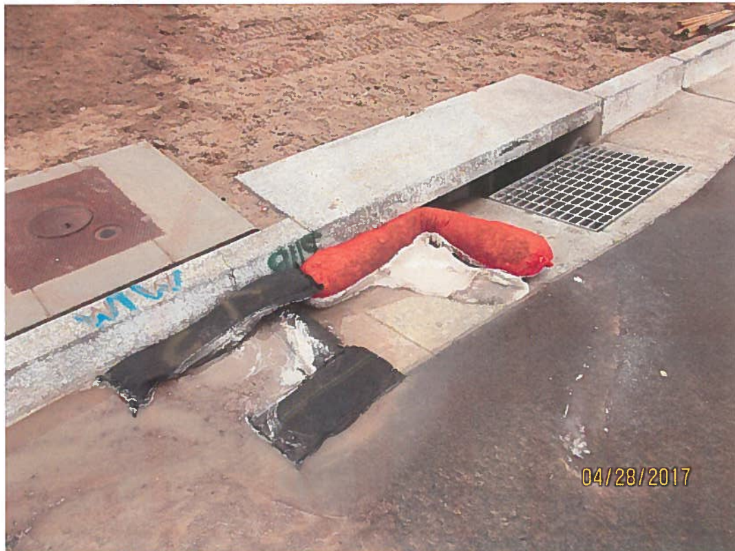
The City placed a rock filter bag and filter sock to reduce the amount of foam entering the arroyo.
