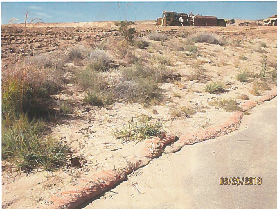
North edge of site showing ineffective sediment BMP.
