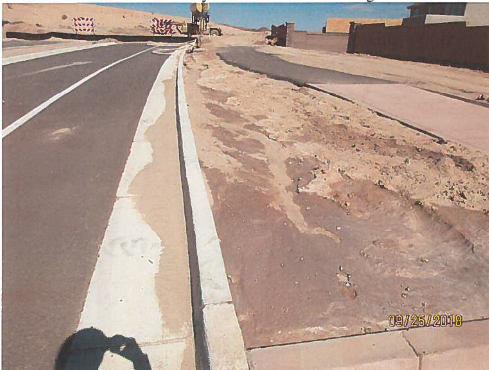
Sediment and/or erosion BMP required in this location at downhill end.
