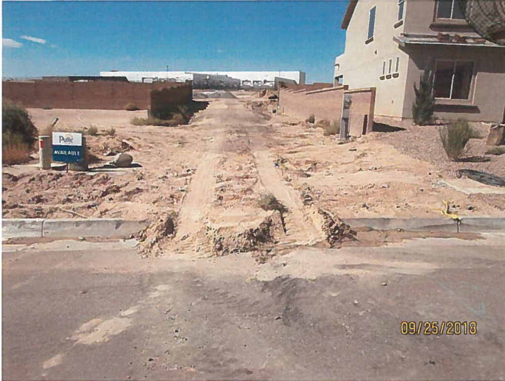
Dirt ramp in street, drainage conveyance with no sediment BMP and no track-out pad.
