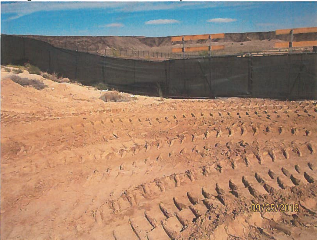
NW corner where pond was filled in. No sediment BMP.
