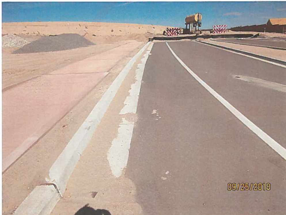
Sediment in Mirehaven Parkway at the south end. South gutter.
