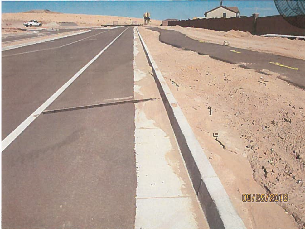
Sediment in Mirehaven Parkway at the south end. North gutter.
