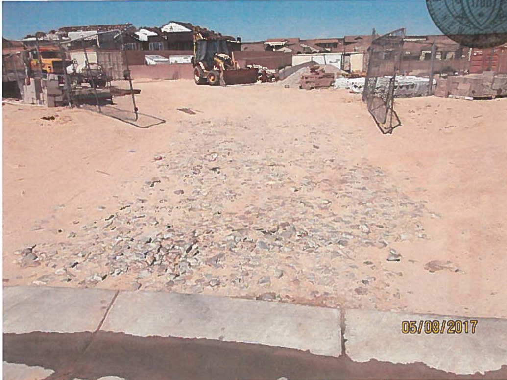
Track-out pad at material storage yard requires maintenance/reinstall.
