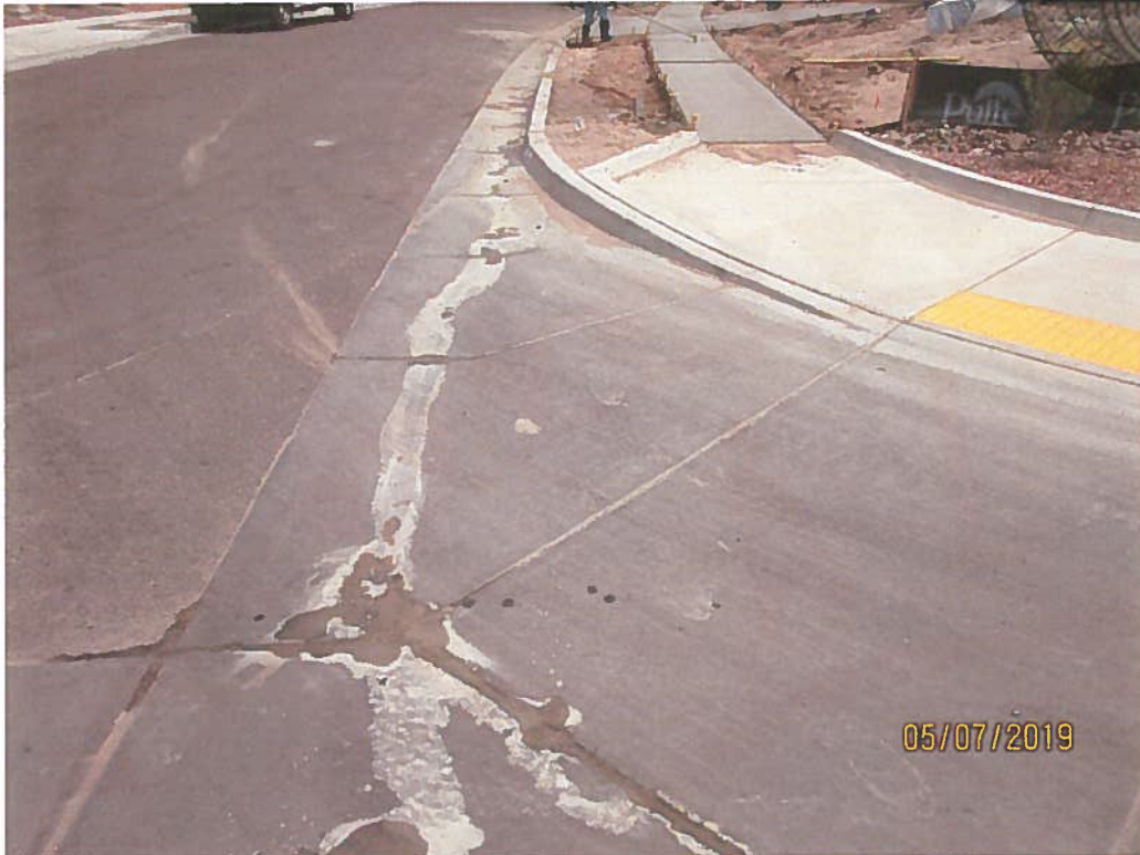
2300 Komatke- concrete slurry running down gutter
