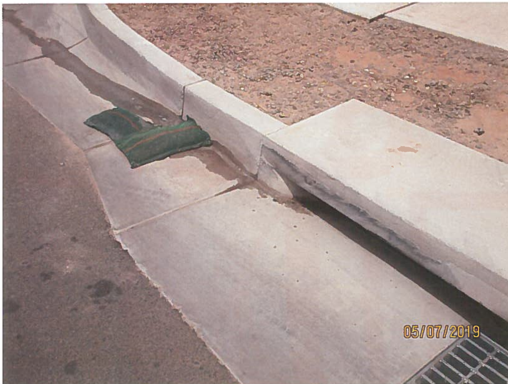
2300 Komatke- concrete slurry entering storm drain inlet
