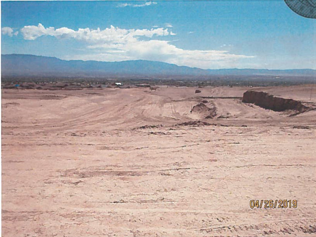
Typical east-west street with no BMP to minimize velocity.
