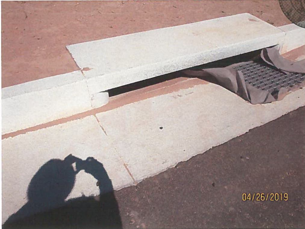
Sediment entering throat of inlet.
