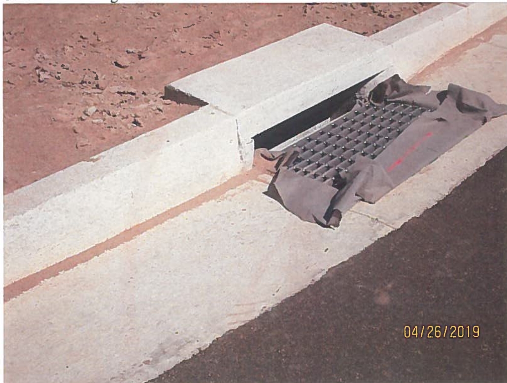
Sediment entering throat of inlet.
