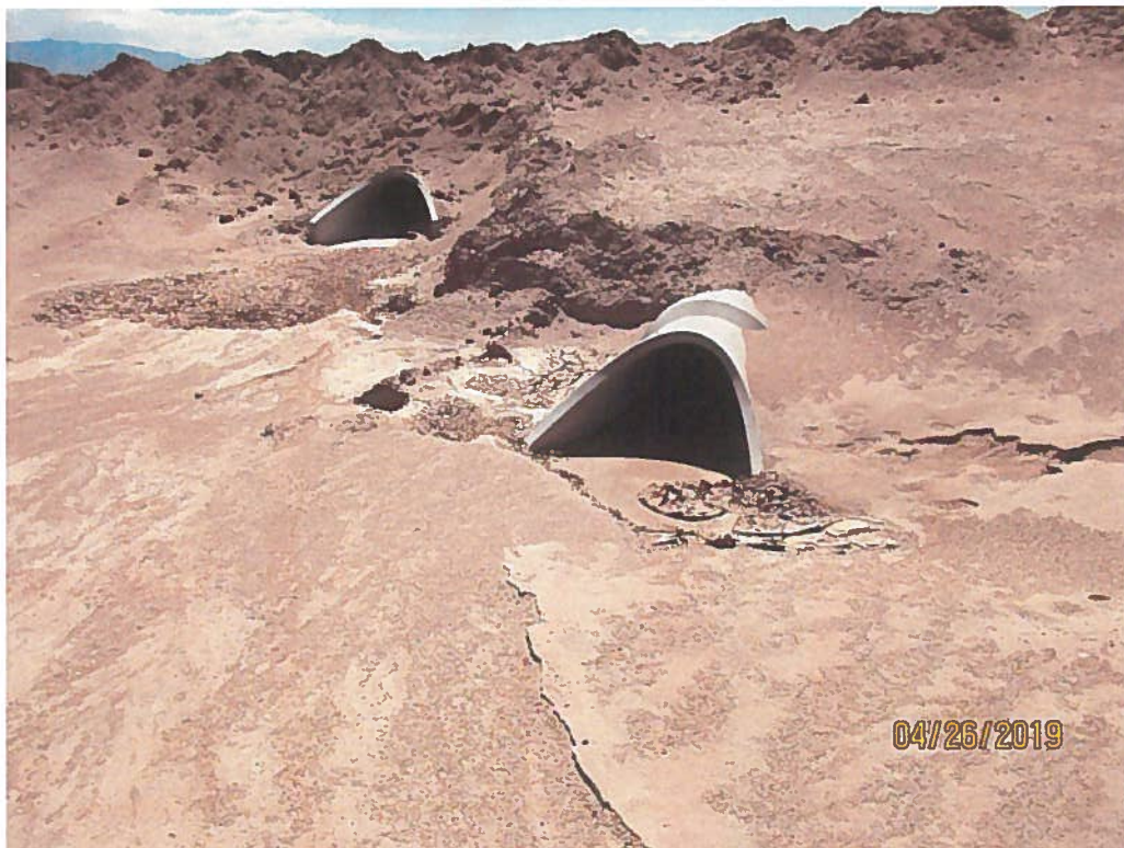
Sediment entering storm drain system. Pond to be re-established.
