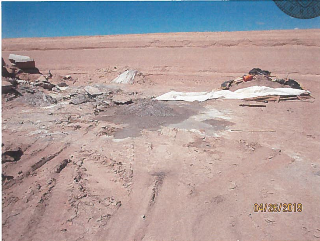
Concrete wash-out on the ground at possible wash-out facility.
