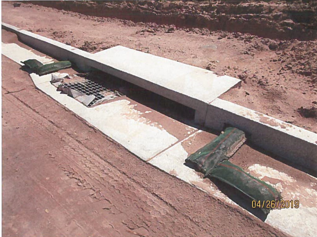
Sediment entering throat of inlet.
