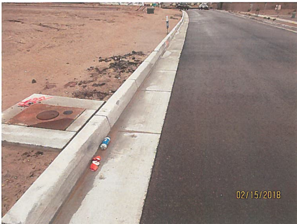
Trash and sediment in gutter on Jet Stream Road.
