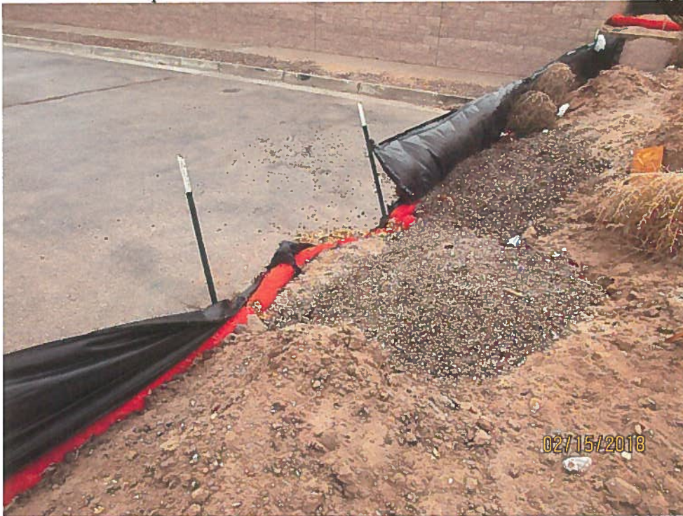
Sediment BMP requires maintenance south end of site at Summer Breeze Dr.
