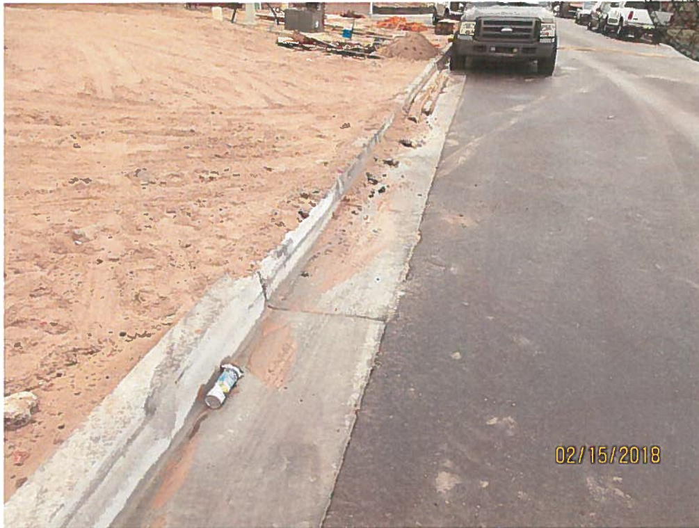
Trash and sediment in gutter on Jet Stream Road.
