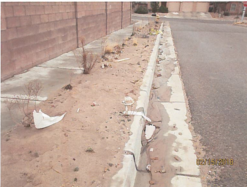
Trash in Animas Place ROW north of project. Sediment in gutter downstream from lot with inadequate cutback.
