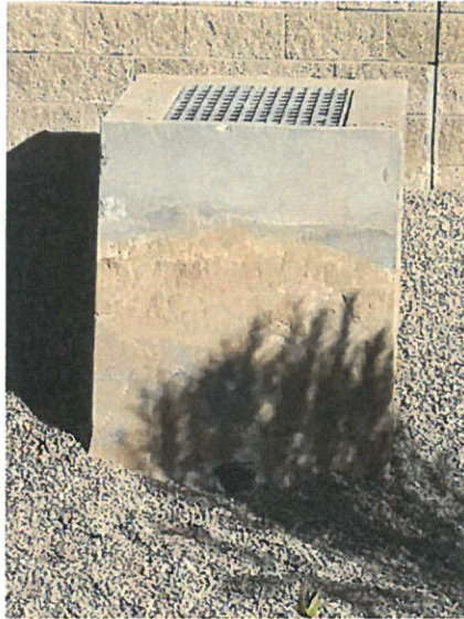
Outfall Structure – Pond 1
