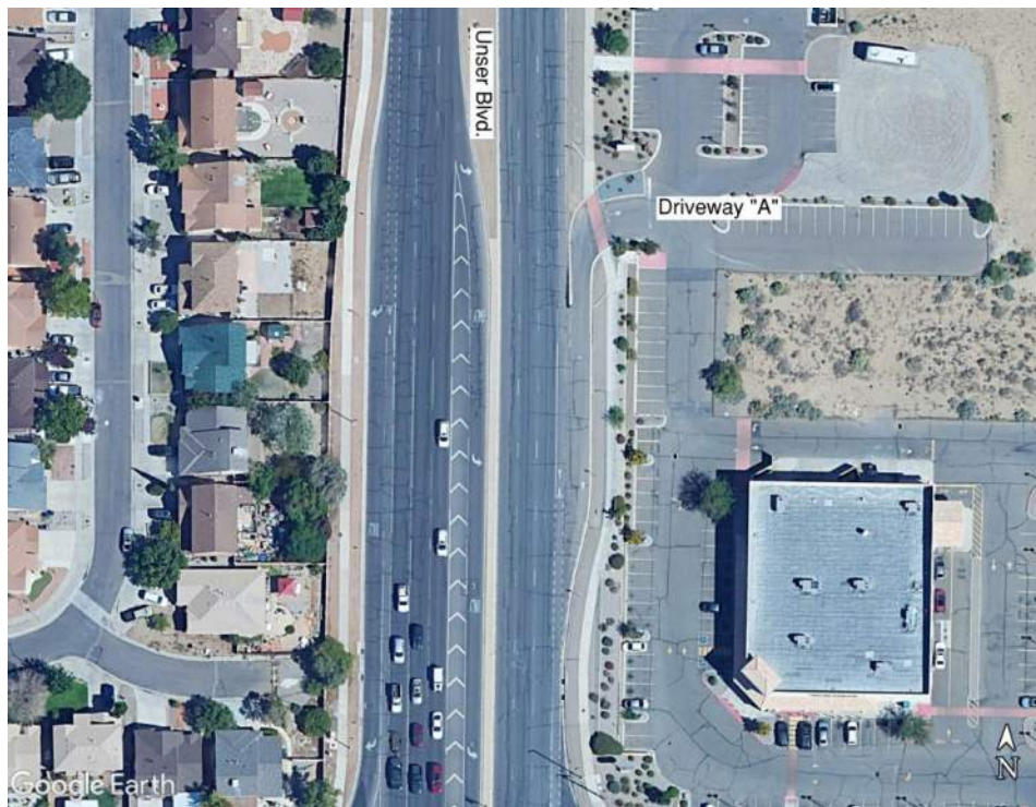
Figure 20 - Aerial Image: Intersection #3
