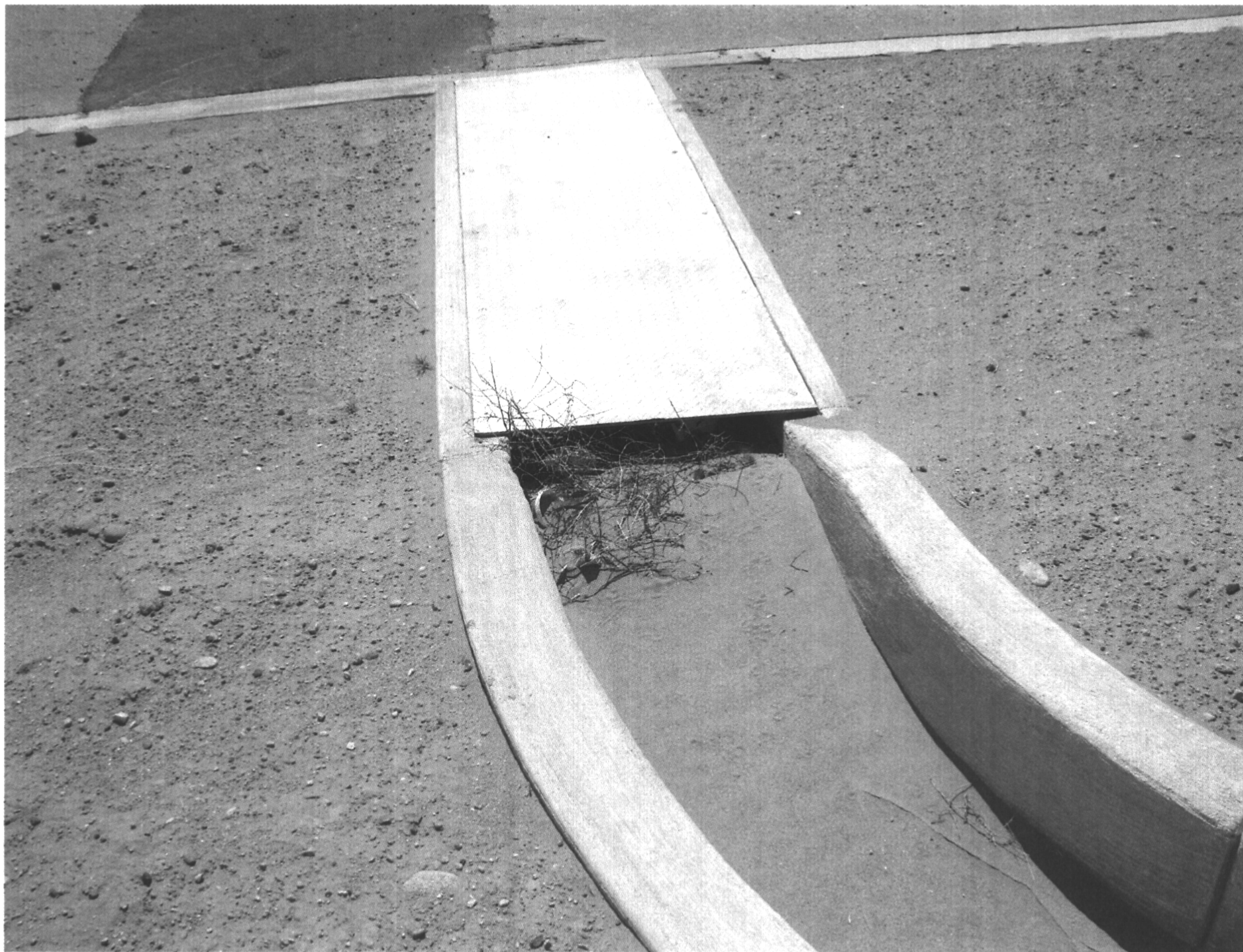
Plugged sidewalk culvert
