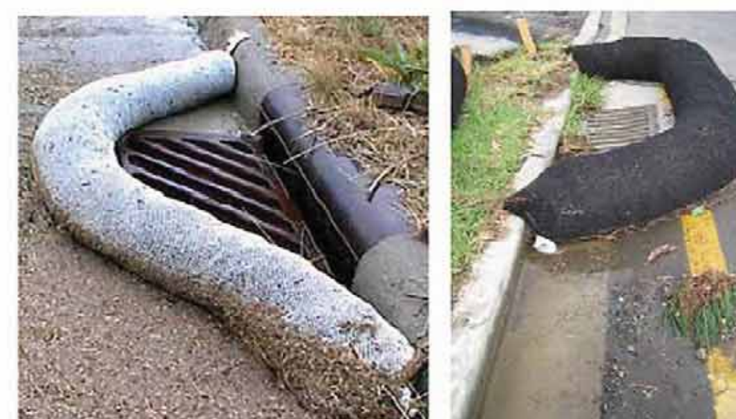
Curb Storm Inlet Protection with Wattles
