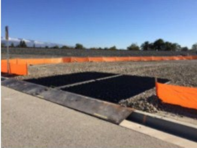
SEDIMENT TRACK OUT CONTROL
