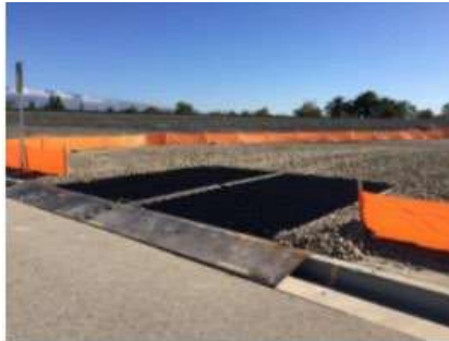
SEDIMENT TRACK OUT CONTROL
