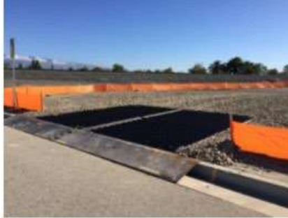
SEDIMENT TRACK OUT CONTROL
