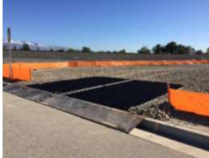
SEDIMENT TRACK OUT CONTROL
