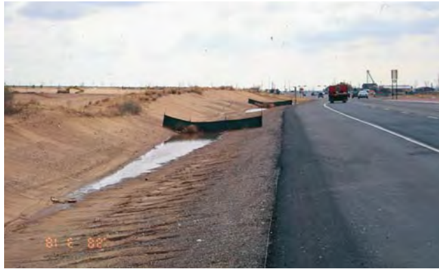
Check dams at roadside ditch
