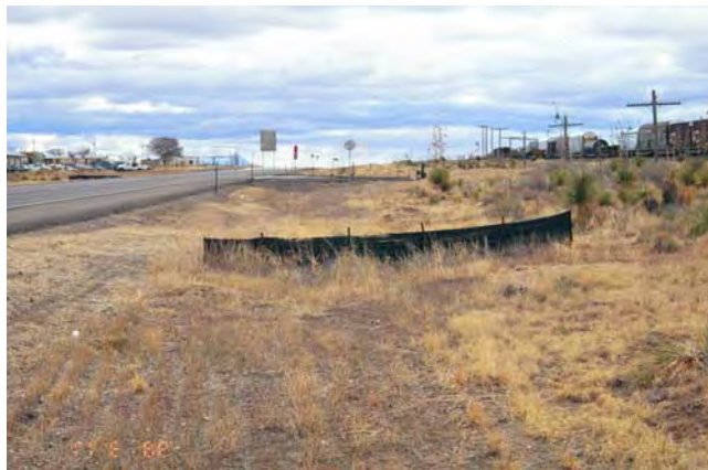
Check dam at roadside ditch
