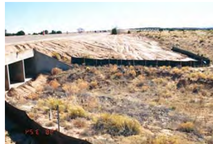
Silt fence at outlet of box
