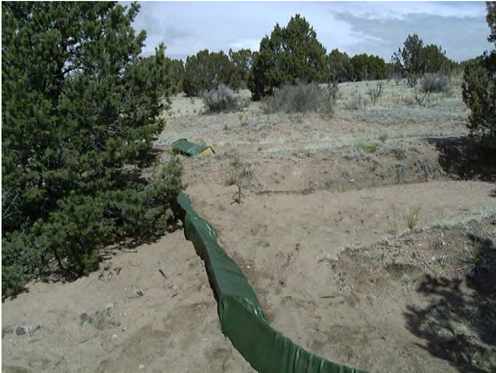
Triangular sediment filter dike
