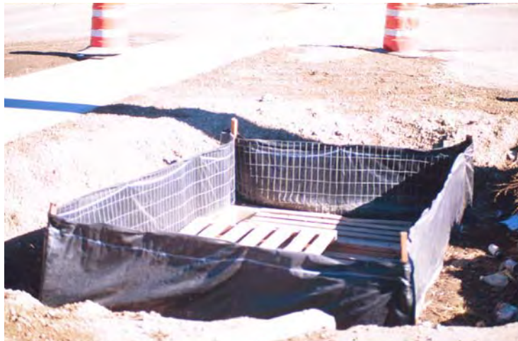
Drop inlet protection in urban area – Type I
