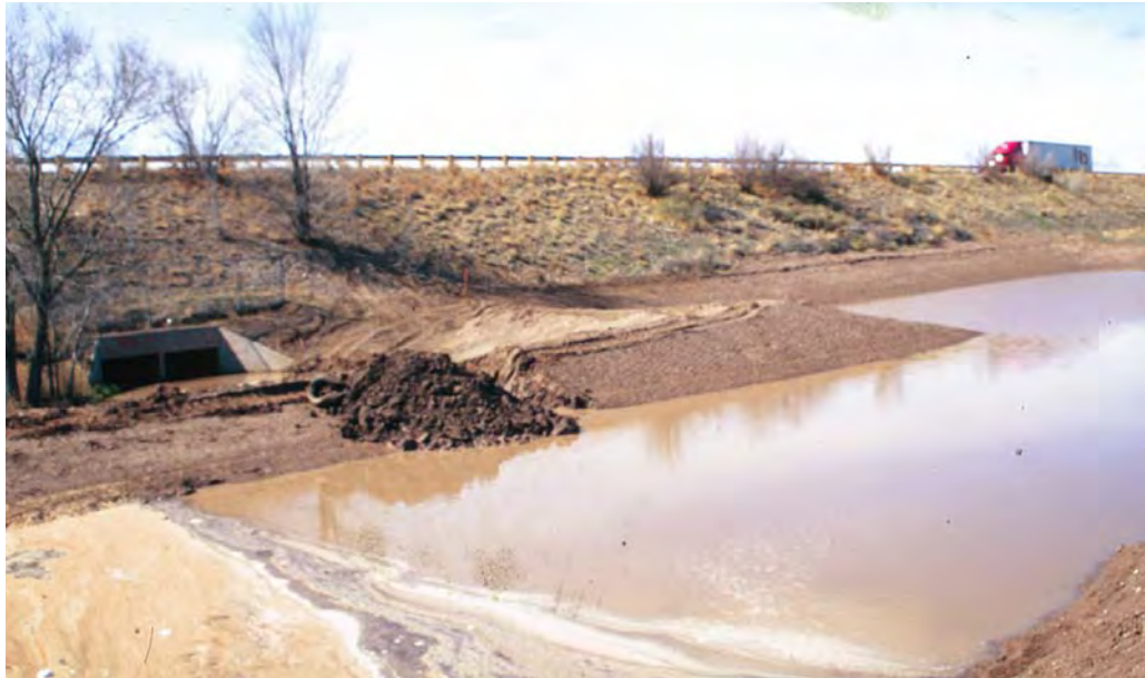
Sediment pond at inlet of box
