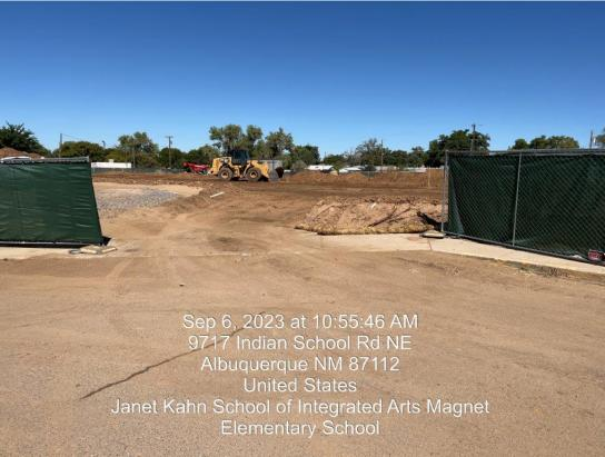
3. **Sediment** was tracked out into the adjacent parking lot where stormwater could easily wash it off into the City's Municipal Separate Storm Sewer System (MS4) and a thin layer of sediment was tracked west several hundred yards from the CE on Indian School Rd. in violation of CGP 2.2.4.d.
