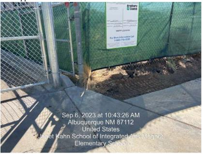
b. the construction exit stabilization (CE) has been missing in violation of CGP 2.2.4 for over a month in violation of the corrective action deadline in CGP 5.2.1.c, and
