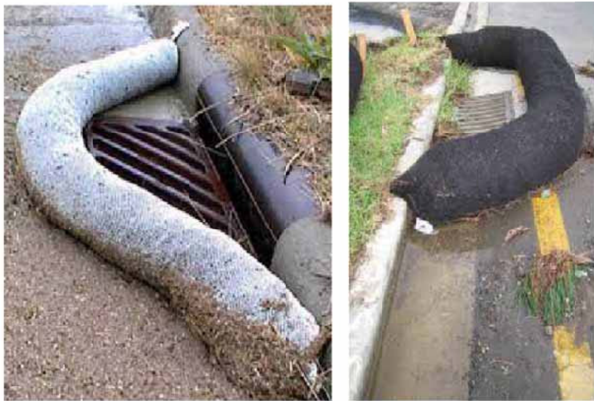
Curb Storm Inlet Protection with Wattles
