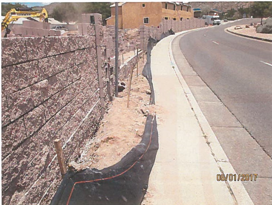
Silt fence and dirt on public sidewalk.
