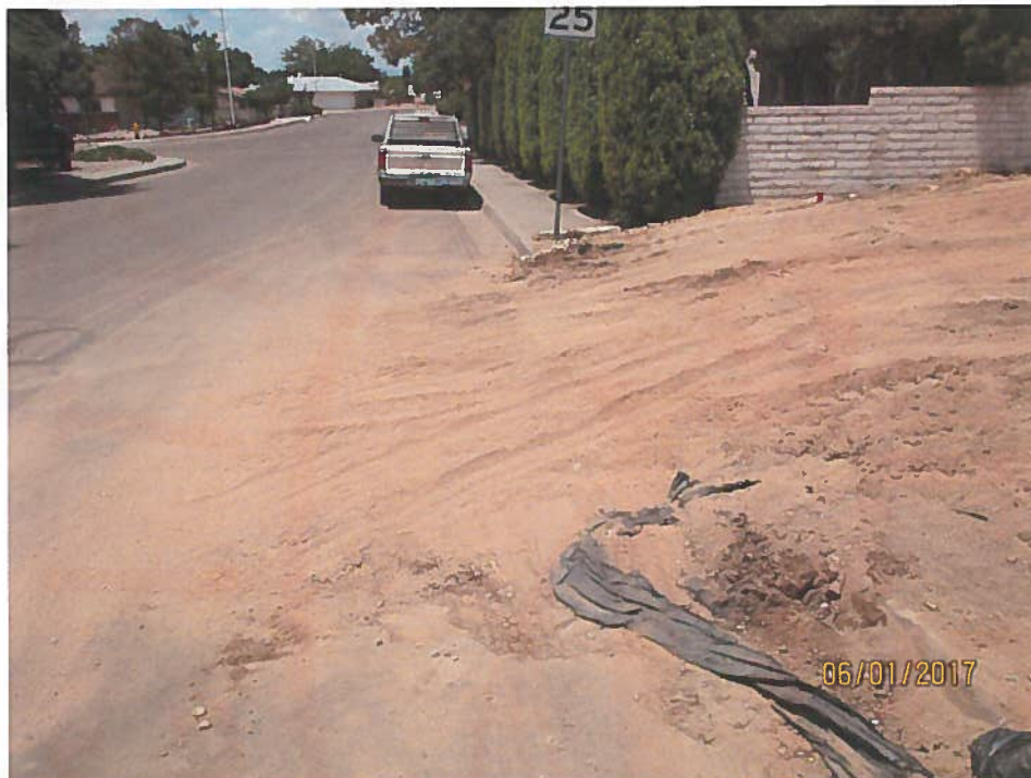
No sediment BMP and large dirt ramp in the street.
