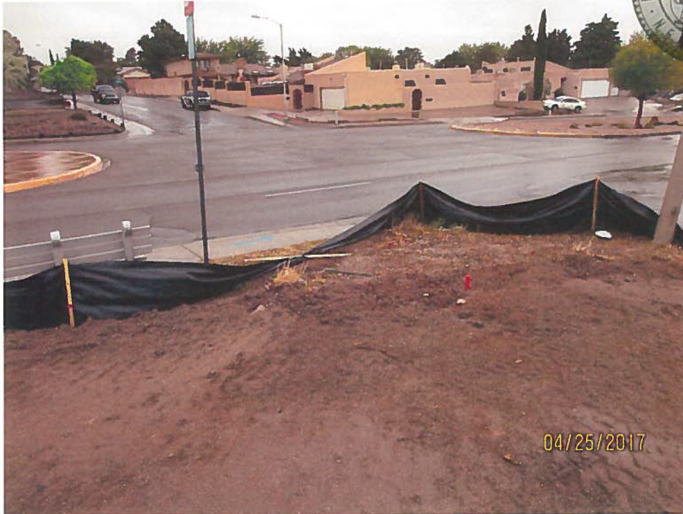
Silt fence in southwest corner. No berm.
