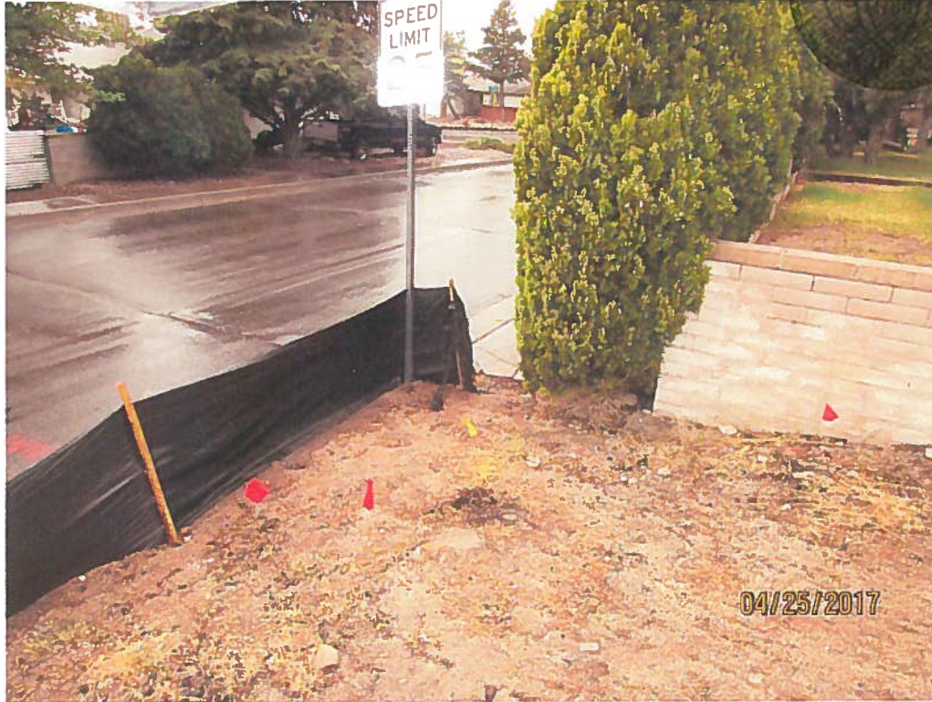
Gap in NW corner. No berm.
