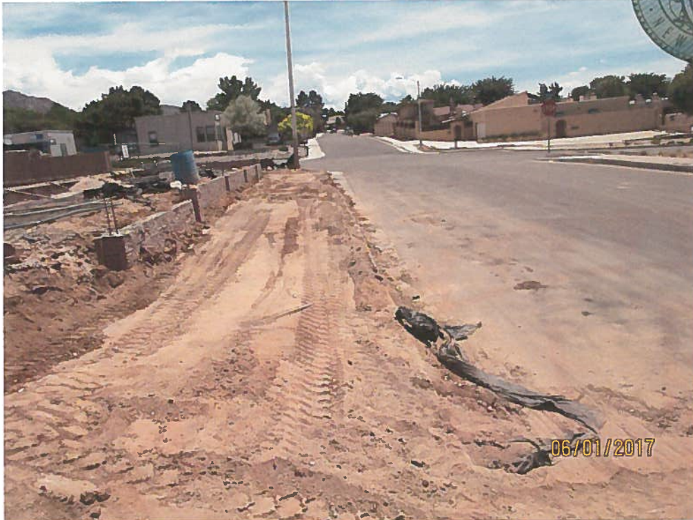
No sediment BMP/silt fence.
