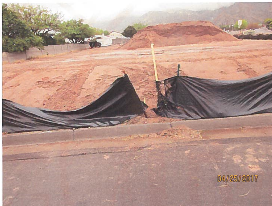
Gap in silt fence and silt fence falling down along Marie Park Dr. Dirt straight-graded to edge and no berm. Sediment observed in street.
