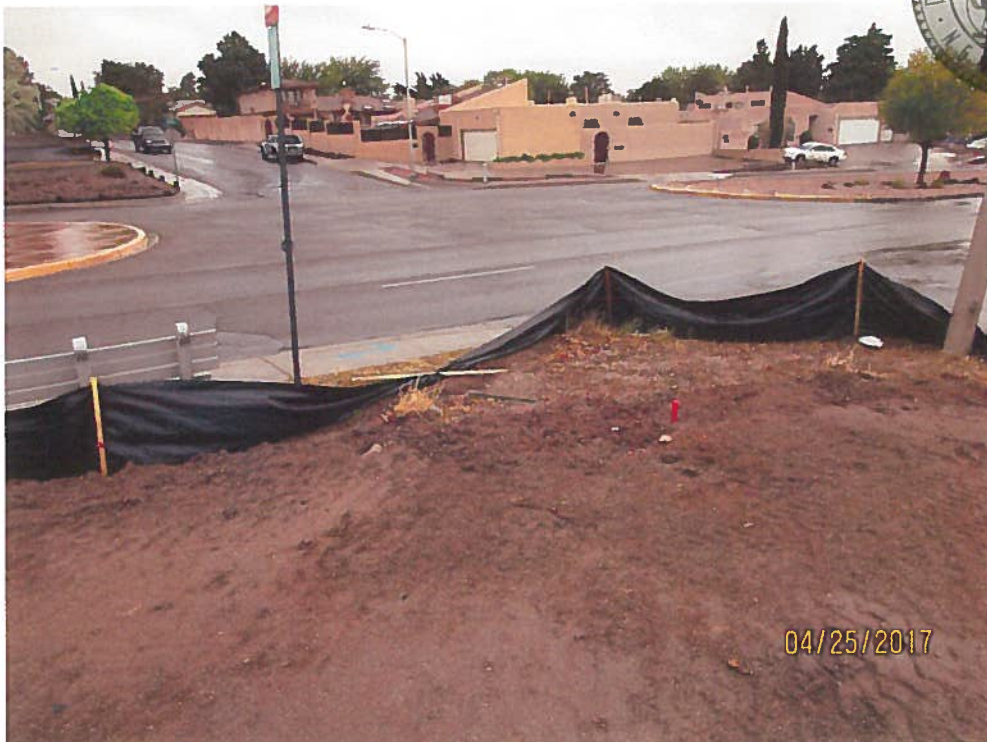
Silt fence in southwest corner. No berm.
