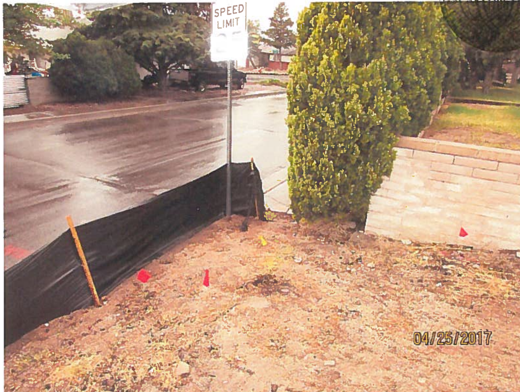
Gap in NW corner. No berm.
