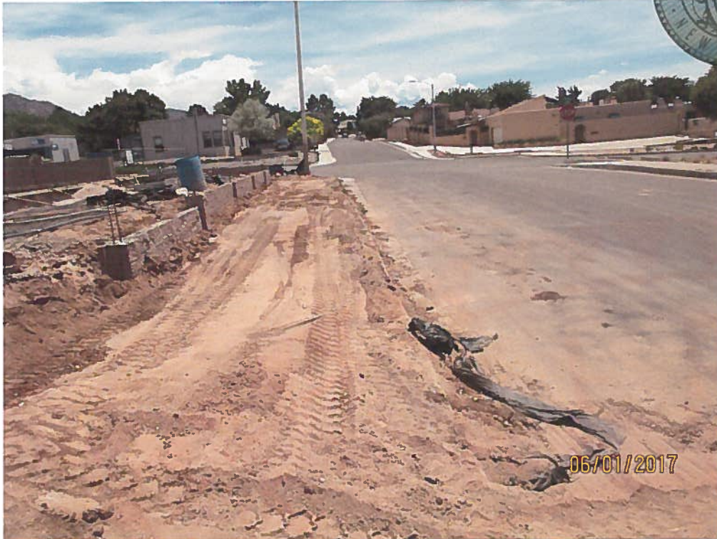
No sediment BMP/silt fence.
