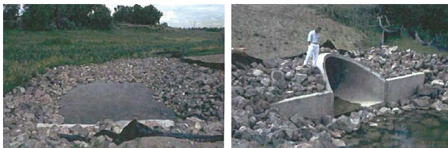
FIGURE 6.11.21 Upstream and Downstream Views of a Low Tailwater Basin in Douglas County
