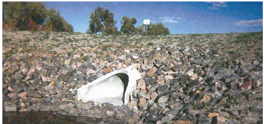
FIGURE 6.11.27 Unprotected Culvert Outlets Cause Downstream Erosion
