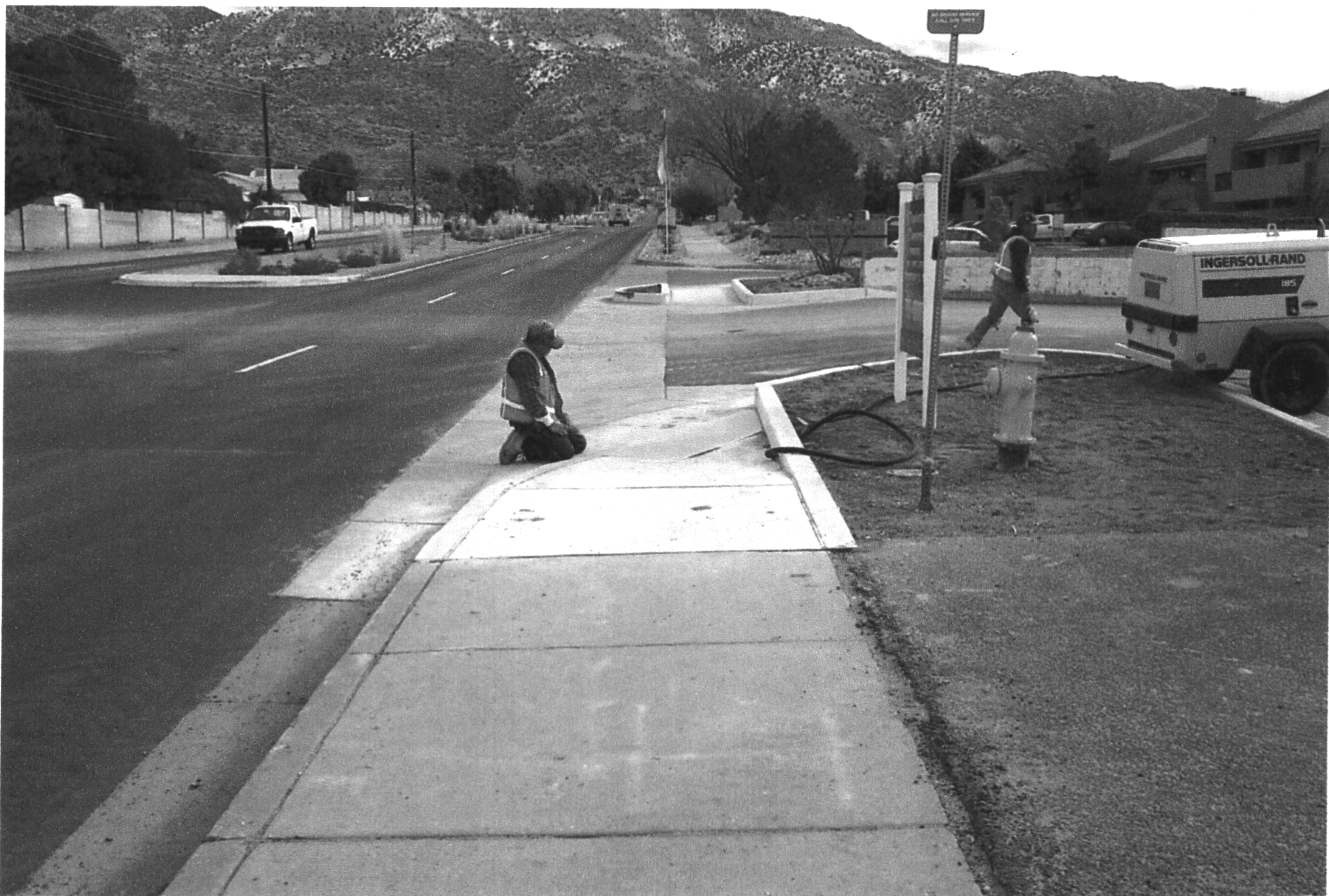
Figure 4. View of truncated dome detectable warning surface being installed in curb access ramp at new entrance to Lot A, Block 31B, Brentwood Hills Subdivision (12/19/07).
