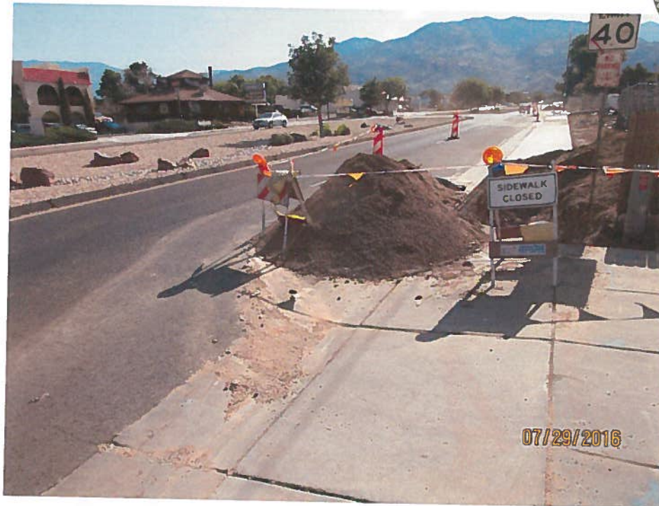
No sediment BMP downstream of dirt pile.
