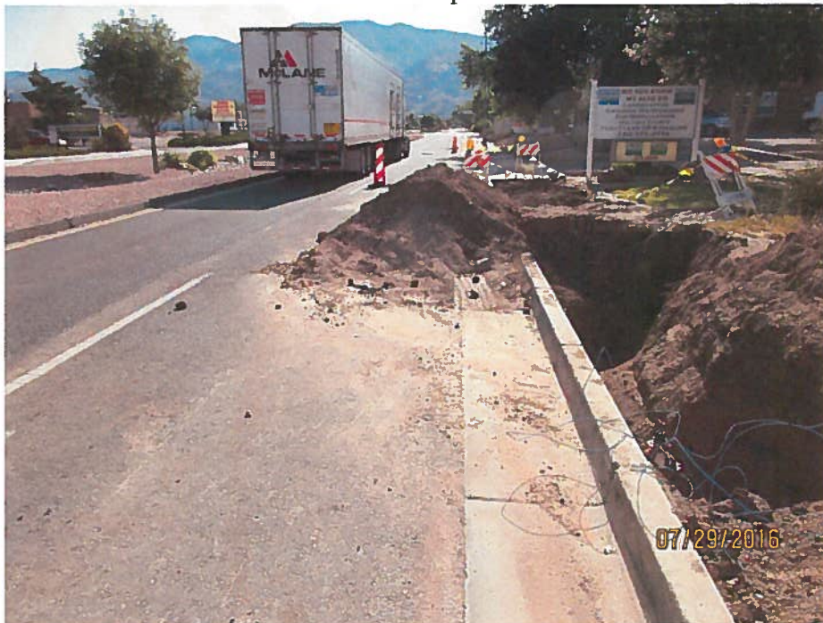
Second dirt pile in Menaul Blvd. No sediment BMP downstream.
