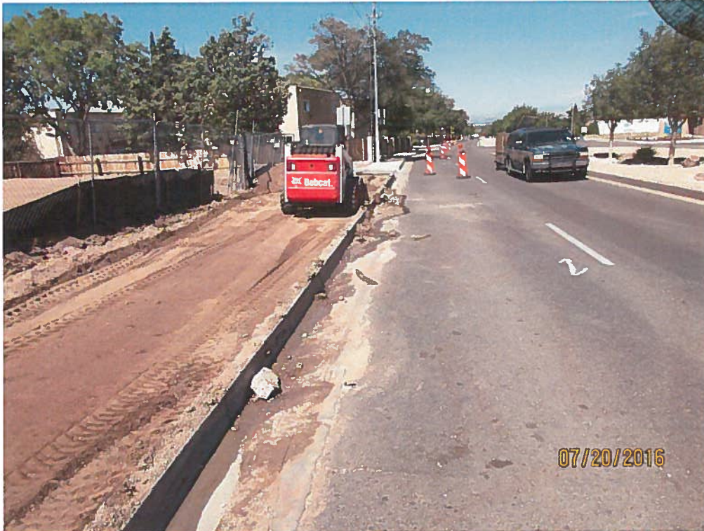
Sediment in Menaul Blvd and water introduced by contractor 7-20-16.
