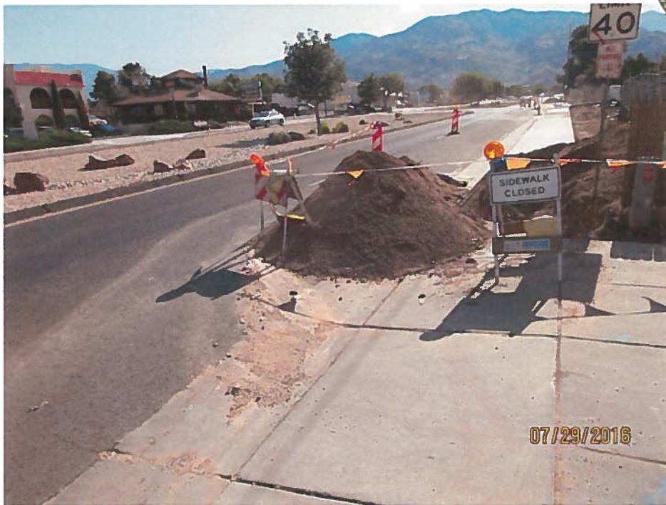
No sediment BMP downstream of dirt pile.
