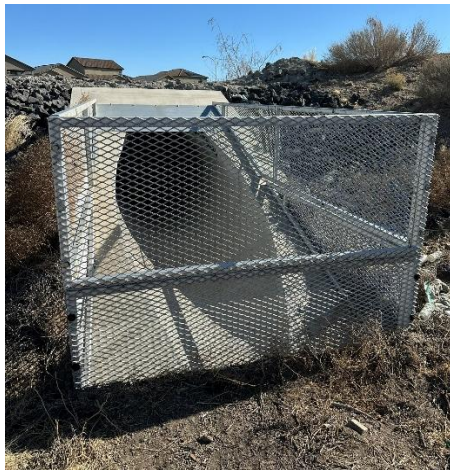
Photo 3: Existing WAHL Pond 60" Orifice Plate Outfall
