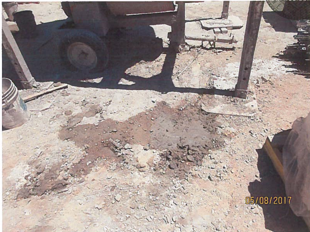
Close-up of cement pollution below large mixers.
