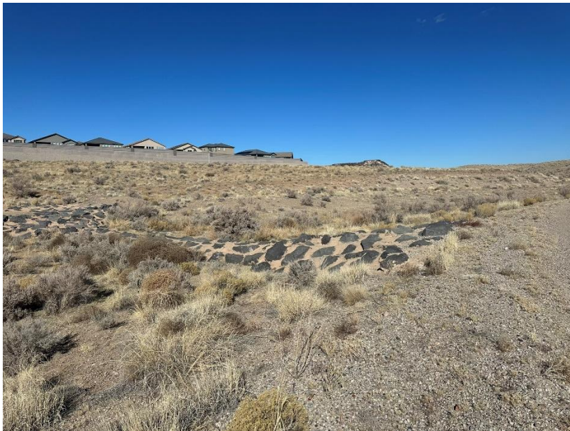
PHOTO 2: CHECK STRUCTURE UPSTREAM OF 54-INCH CULVERT
