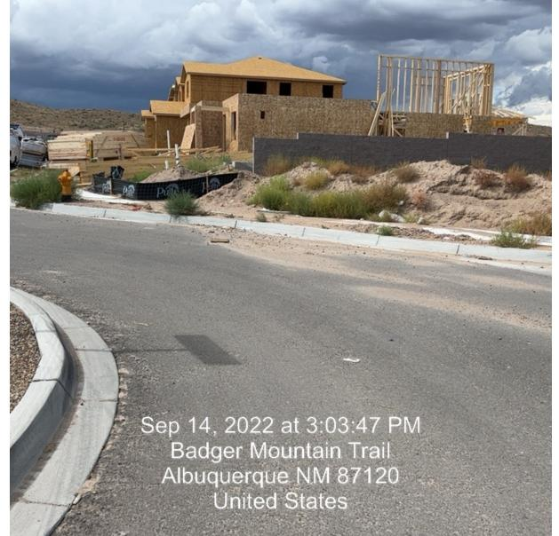
Silt Fence repairs, replacement, and additions are needed in several locations along the northern perimeter. Additional Silt fence is needed at the above photo of Badger Mountain Trail.
