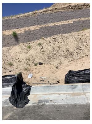
**Deficiency Name:** Soda springs **Corrective Actions:** Repair or replace damaged silt fence in multiple areas along Soda Springs
