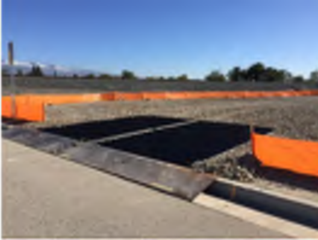
SEDIMENT TRACK OUT CONTROL
