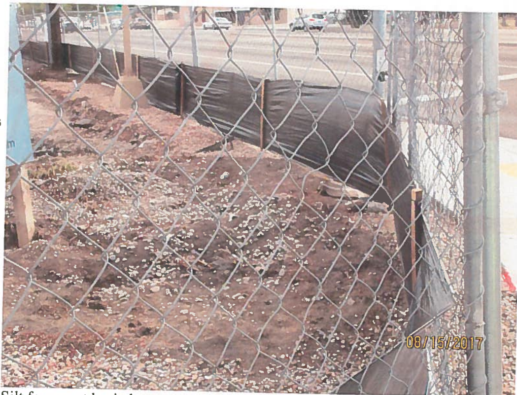
Silt fence not buried.
