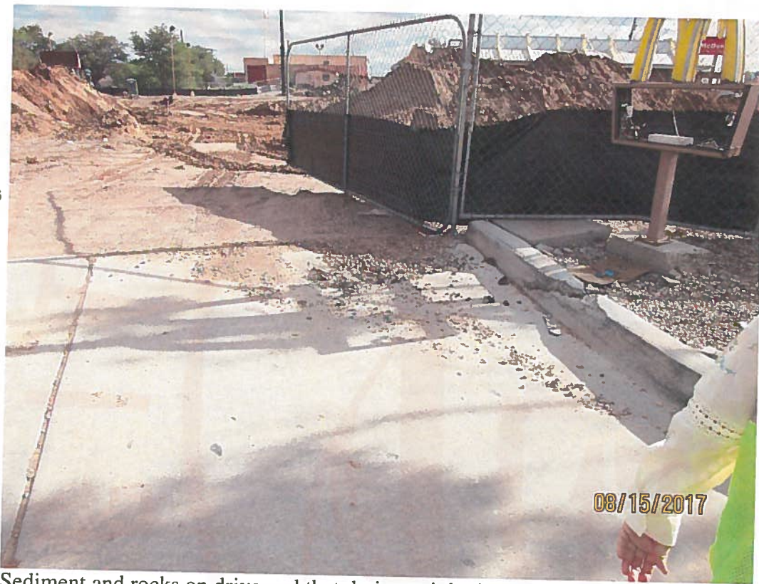
Sediment and rocks on drive pad that drains to inlet in Hanover St.
