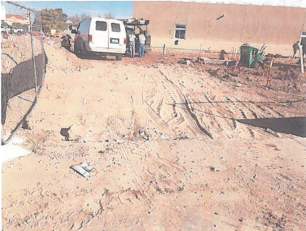
No track-out pad and track-out onto drive pad.
