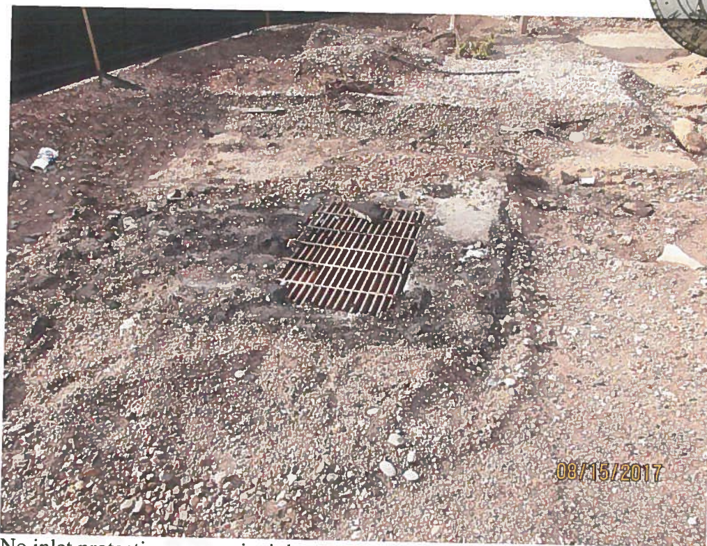
No inlet protection on on-site inlet.
