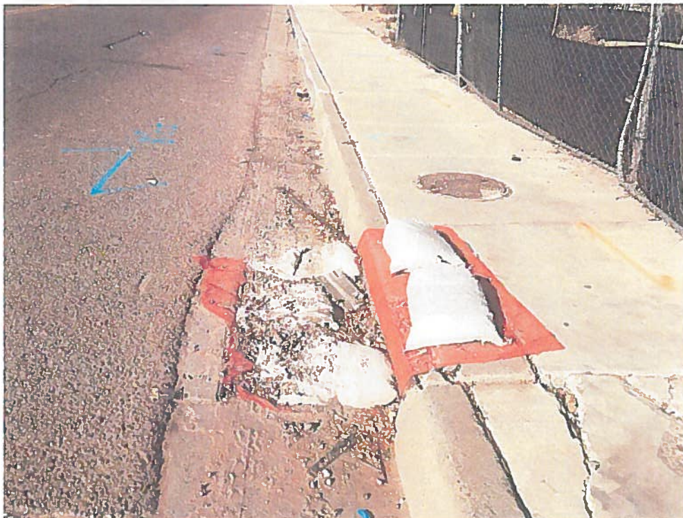
Inlet protection requires maintenance and sediment in gutter.
