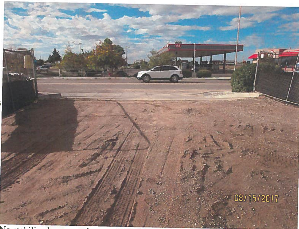
No stabilized construction entrance.
