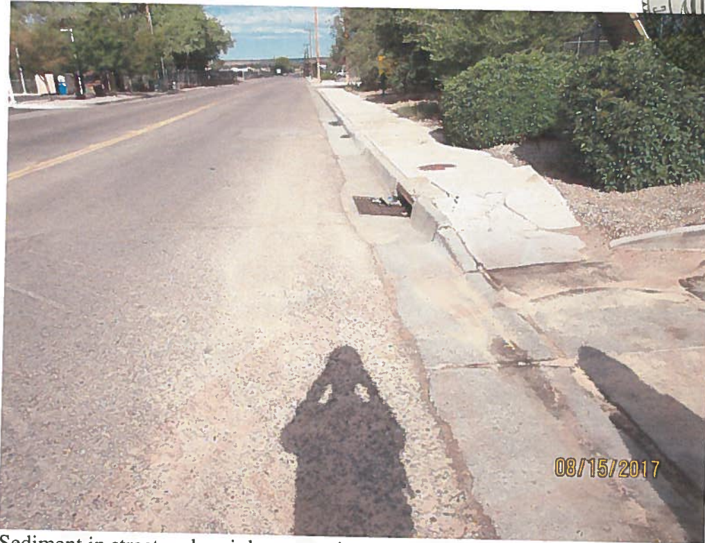
Sediment in street and no inlet protection.
