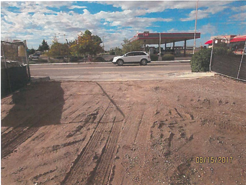
No stabilized construction entrance.
