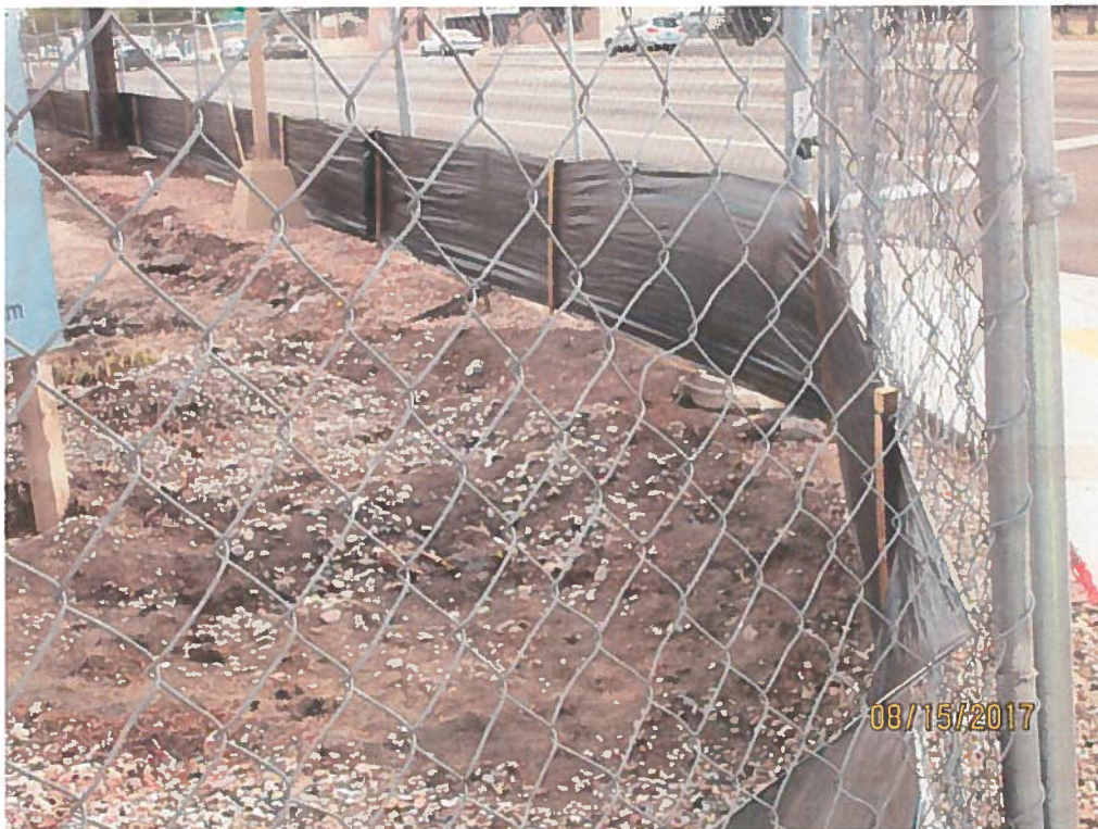
Silt fence not buried.
