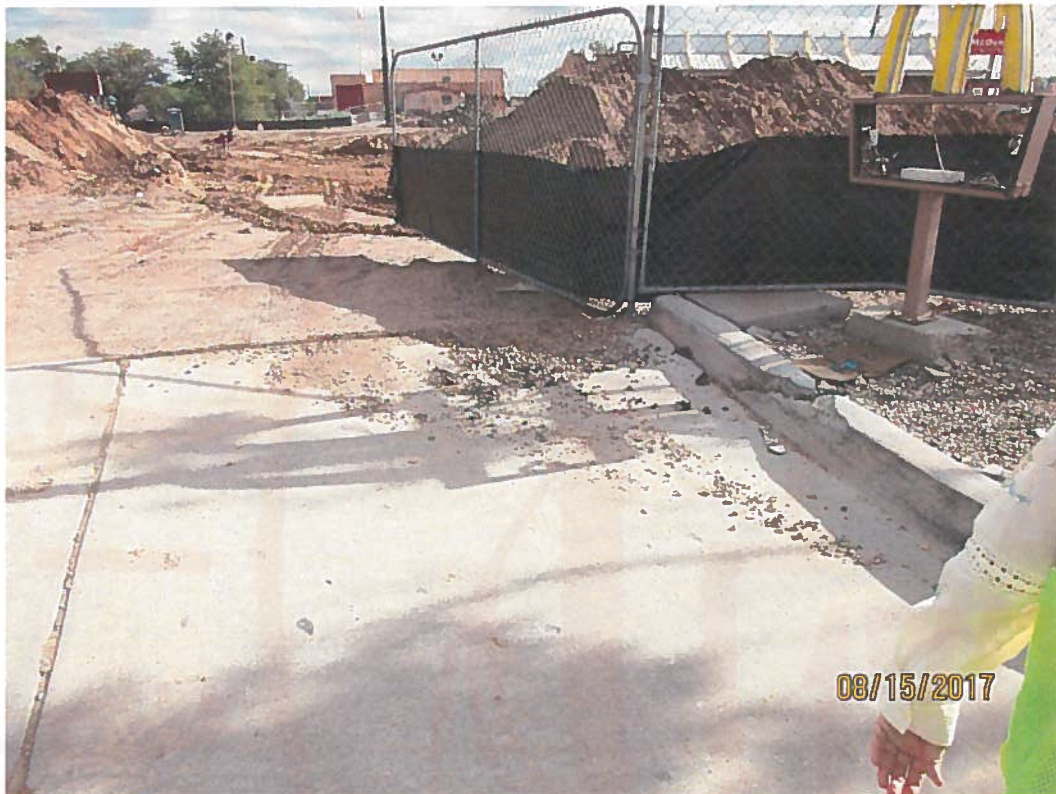
Sediment and rocks on drive pad that drains to inlet in Hanover St.
