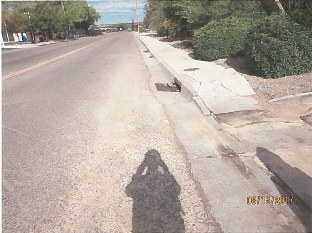
Sediment in street and no inlet protection.
