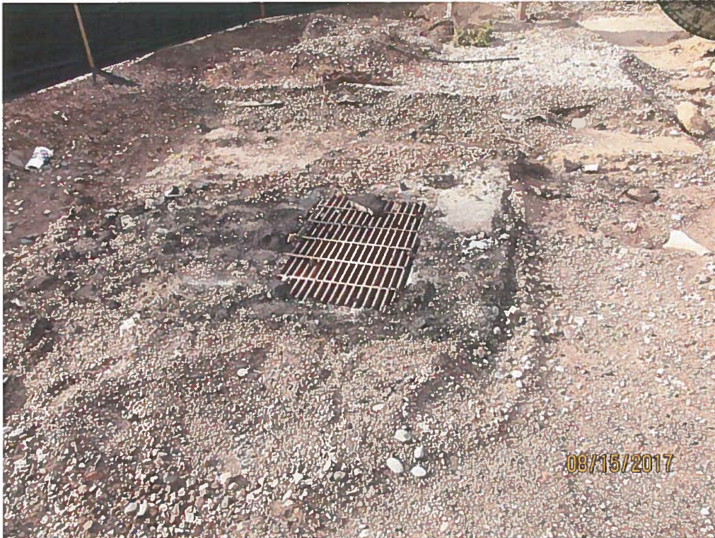
No inlet protection on on-site inlet.
