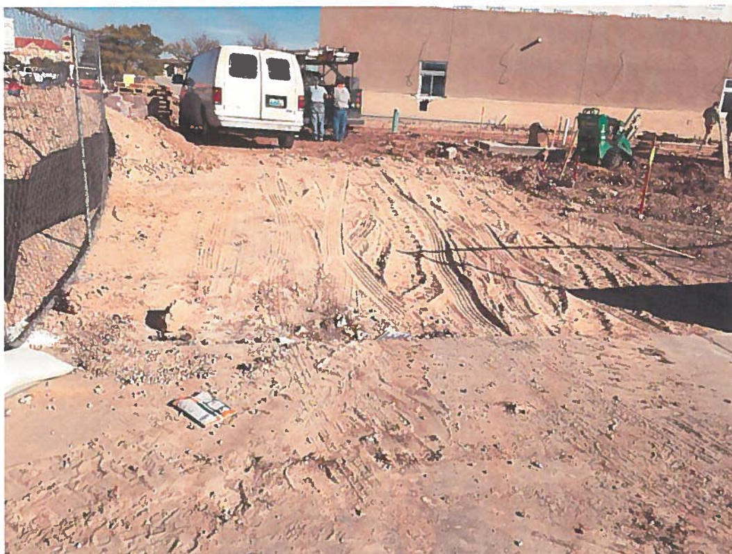
No track-out pad and track-out onto drive pad. Trash outside project boundary.
