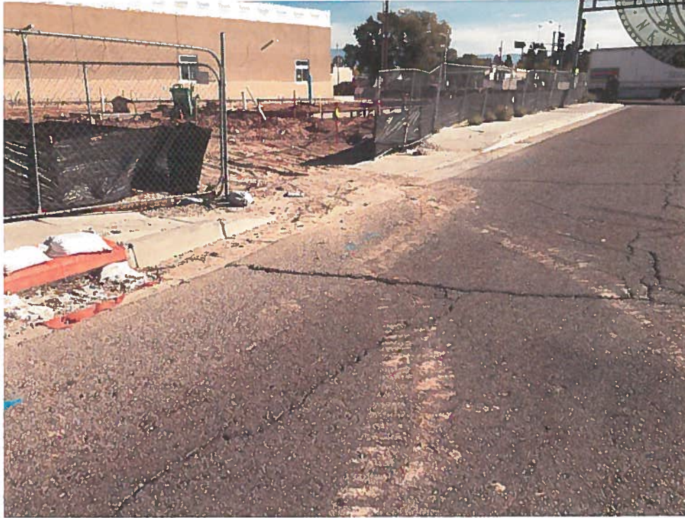
Track-out onto street and sediment in gutter and in street.
