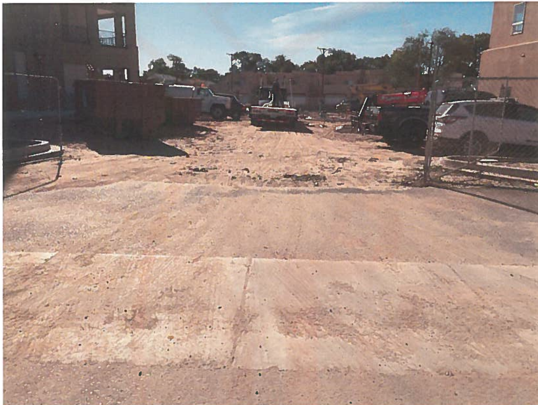
Stabilized construction exit/Track-out pad in poor condition.
