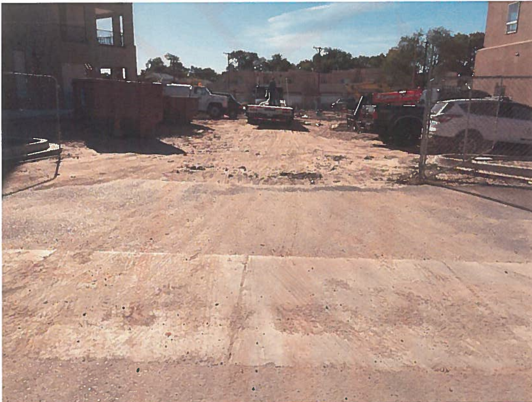
Stabilized construction exit/Track-out pad in poor condition.
