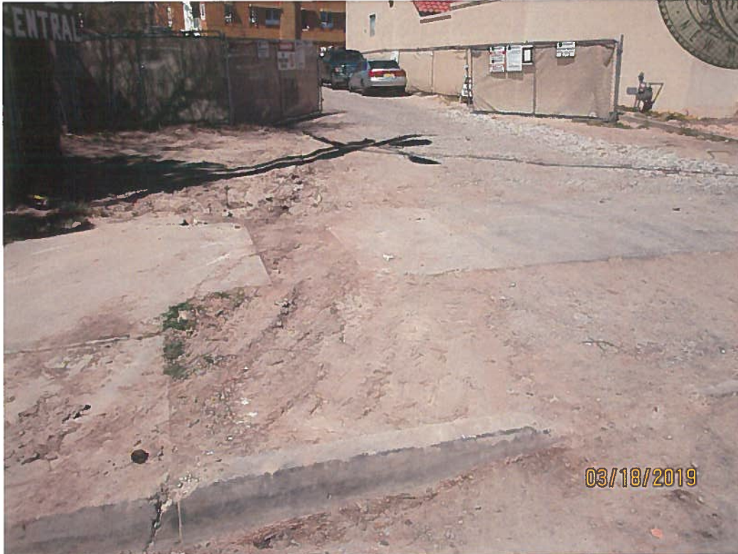
Vehicle tracking control pad requires maintenance.
