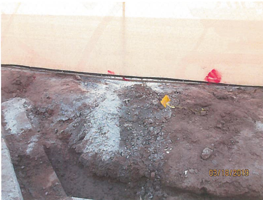
Wash-out in dirt north side of building.
