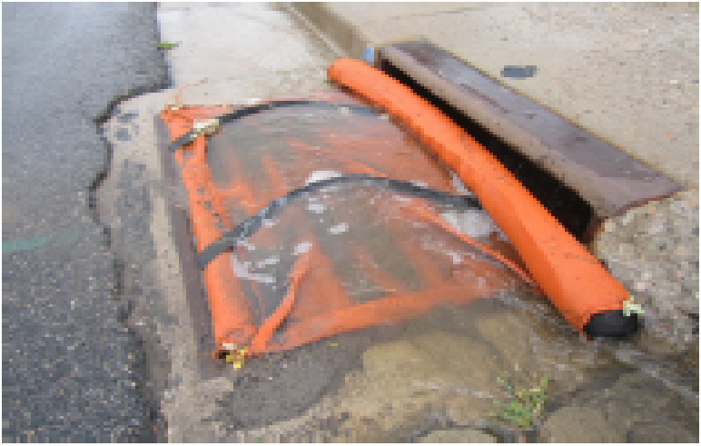
Storm drains and curb inlets should be protected with filter fabric and filter socks, which trap sediment and allow water to flow through. Photo Credit: PG Environmental for USEPA
