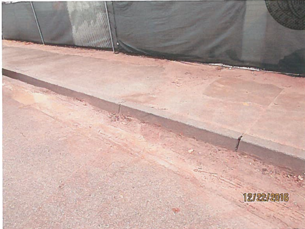
Sediment in gutter on 20 th St. There is a gap in the silt fence in this location.
