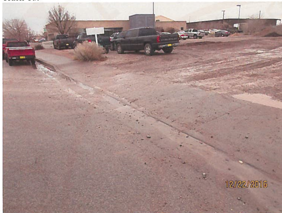
Laydown yard, no track-out pad. Sediment on sidewalk and in gutter.
