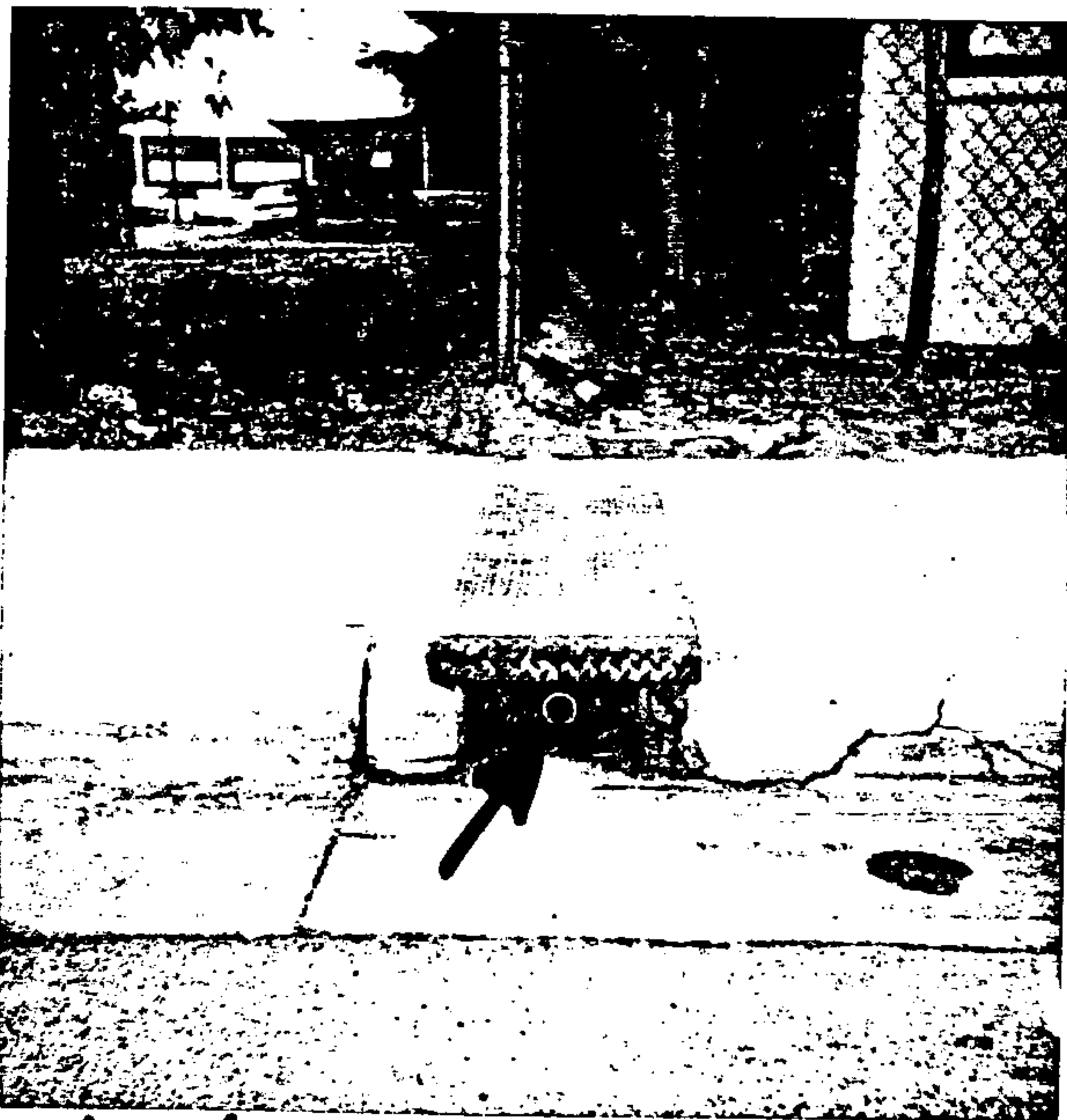
5/15/00 Jaguar P.M. Note new 4" discharge from old SW Culvert
