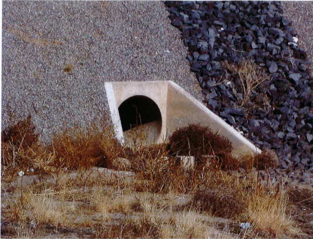
(3) Northeast corner inlet structure
