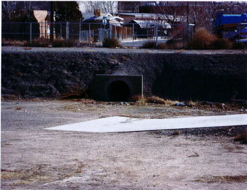
(4) South side inlet structure
