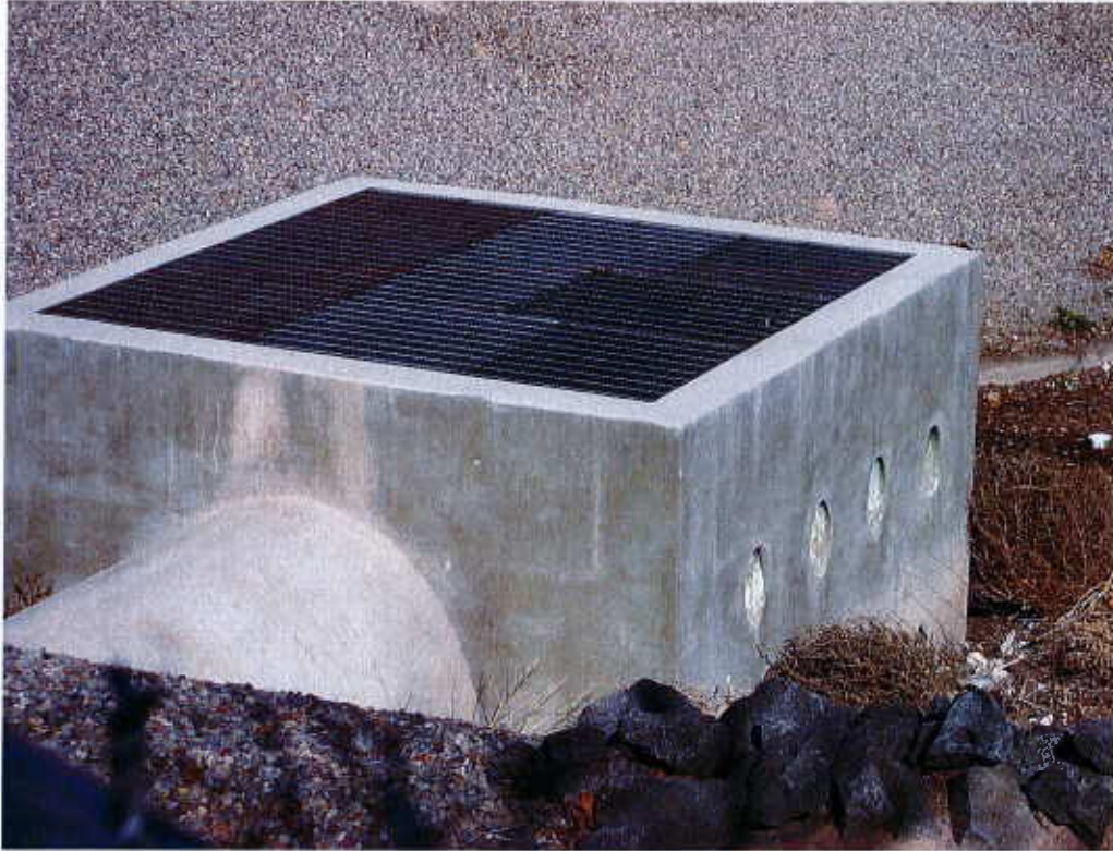
(9) West side principal outlet structure (3)
