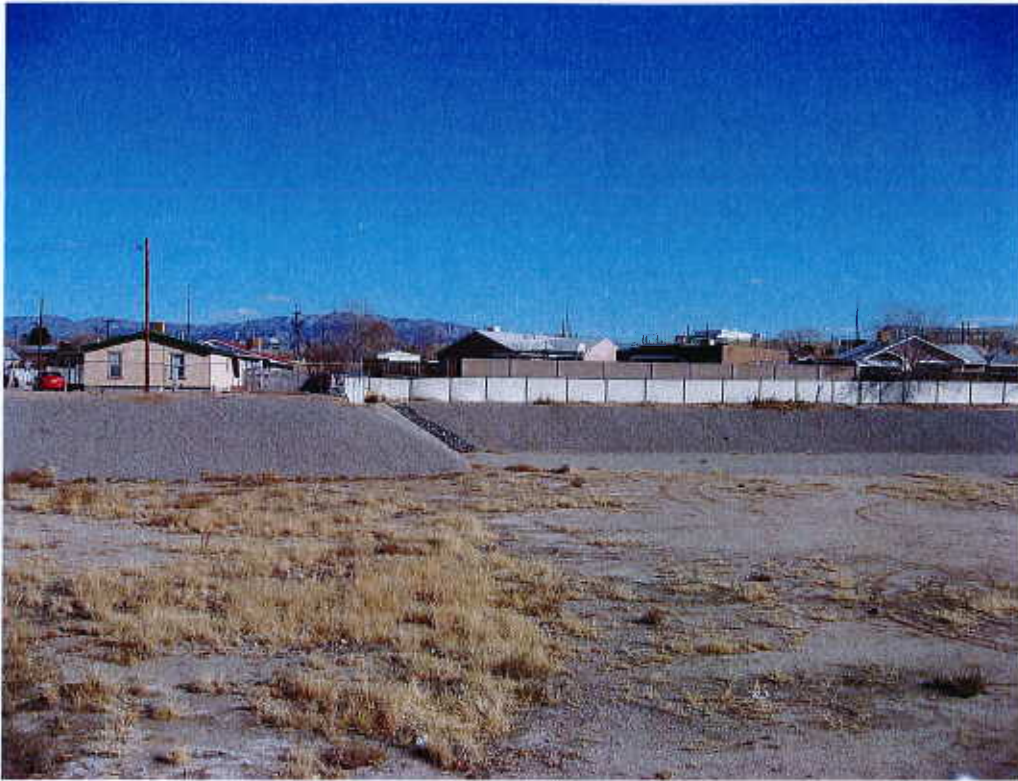
(1) East side of Air Quality Pond
