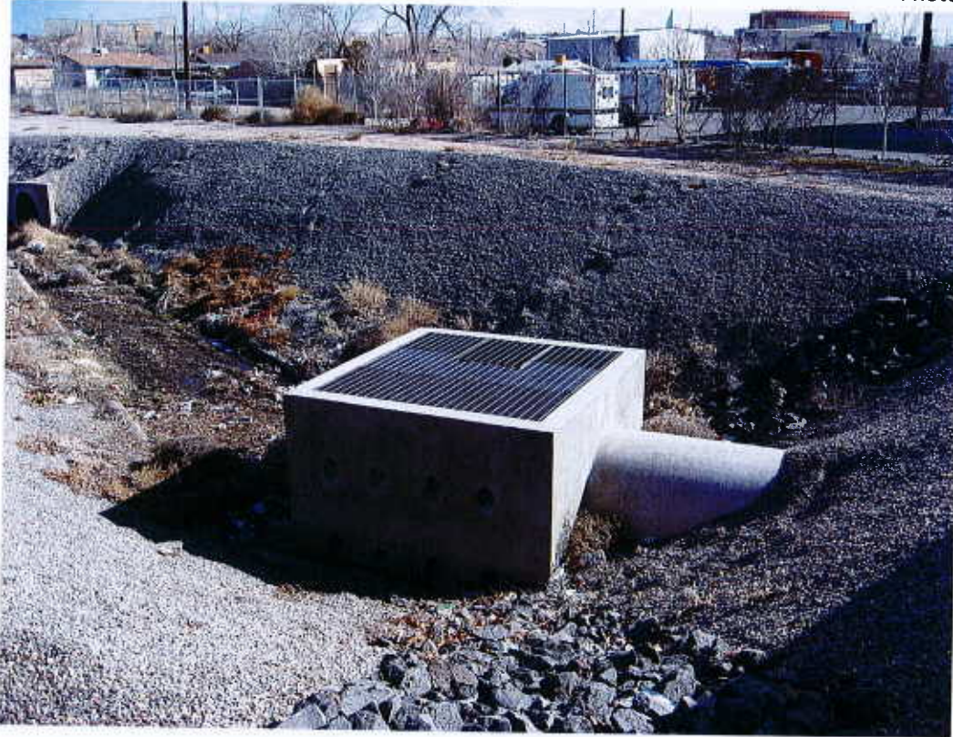
(7) West side principal outlet structure
