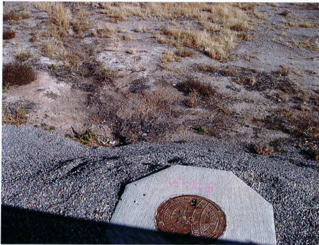
(6) West side outlet structure
