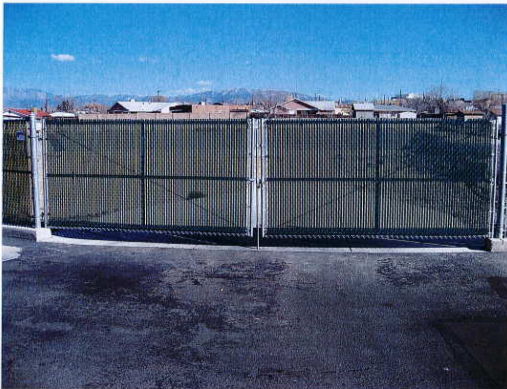
(10) West side ramp
