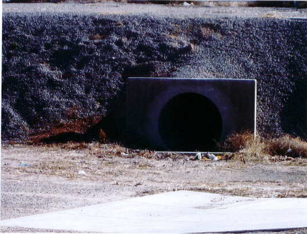
(5) South side inlet structure (2)
