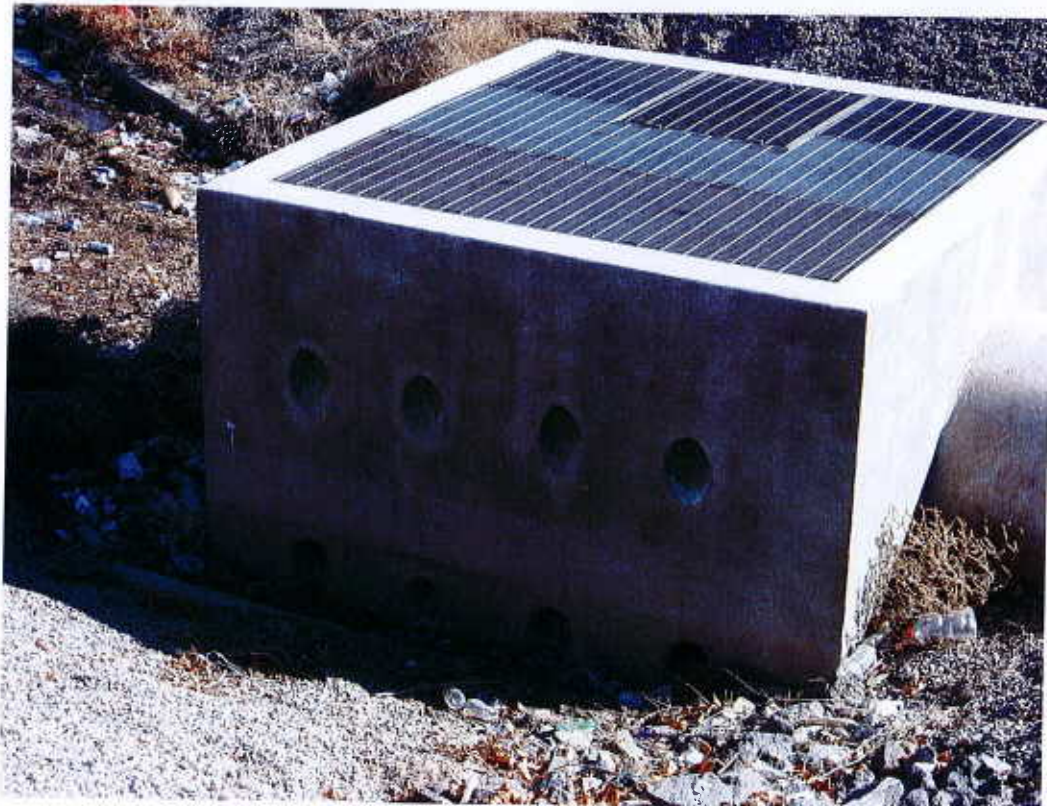
(8) West side principal outlet structure (2)
