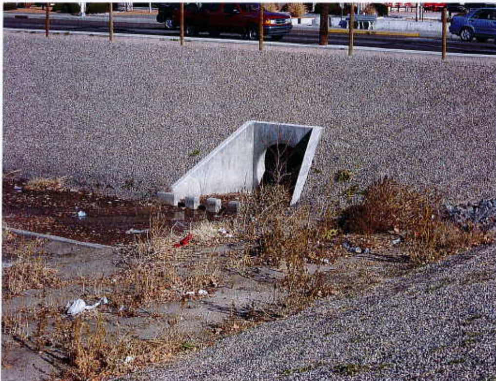
(2) East side inlet structure
