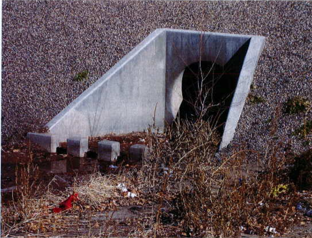
(3) East side inlet structure
