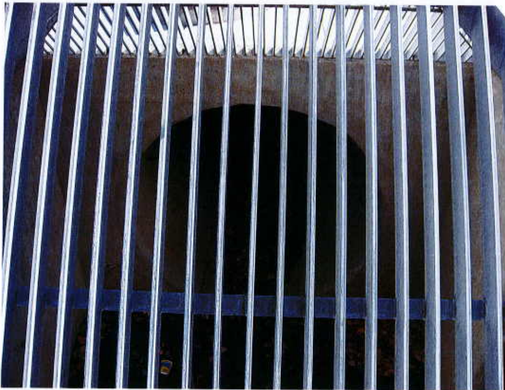
(10) Outlet structure - 96 inch east outlet
