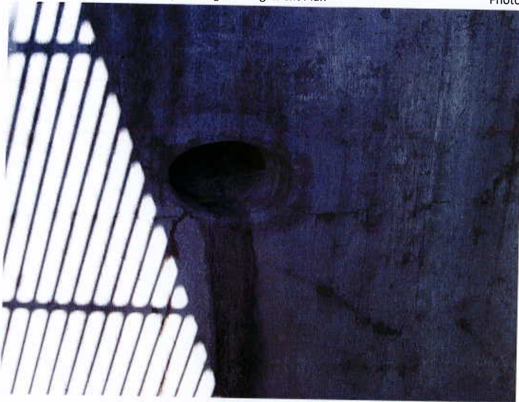
(7) Outlet structure - 12 inch north outlet
