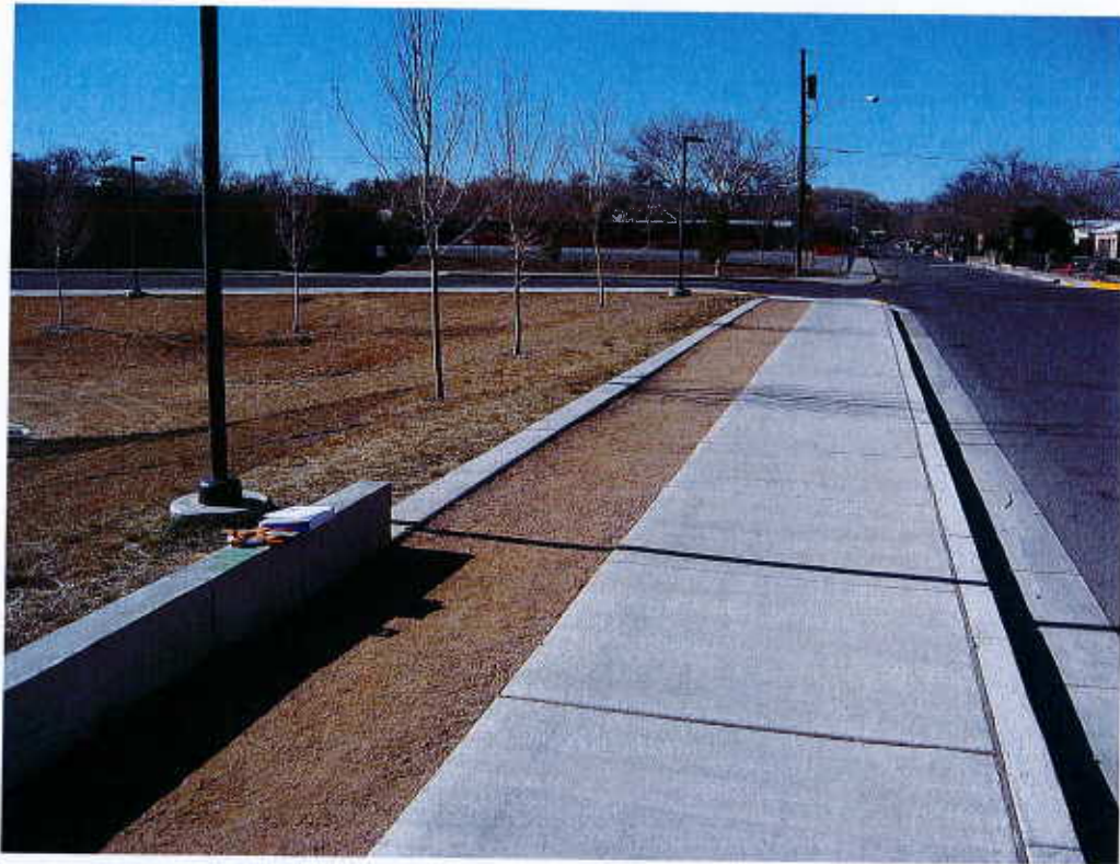
(1) Looking at northwest corner
