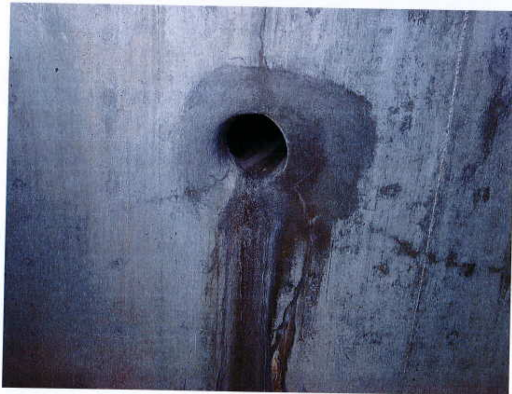
(8) Outlet structure - 12 inch south outlet
