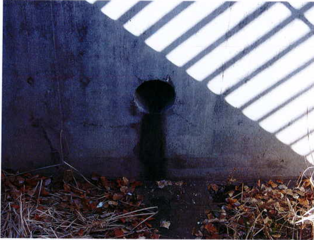
(9) Outlet structure - 12 inch west outlet
