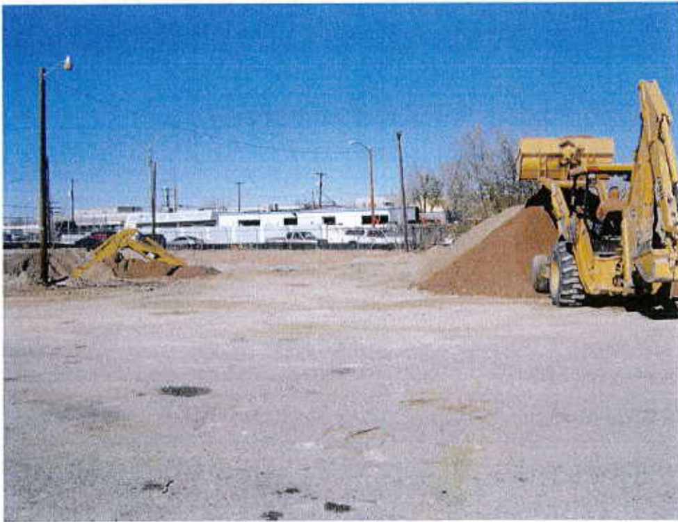
B.14, Segregating Soil with Petroleum Hydrocarbons
