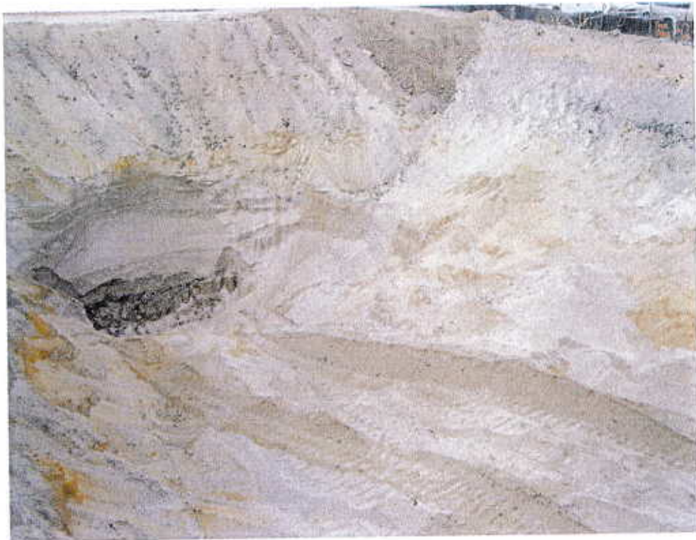
B.5, Soil Benching for Reaching Deeper Contaminated Soil
