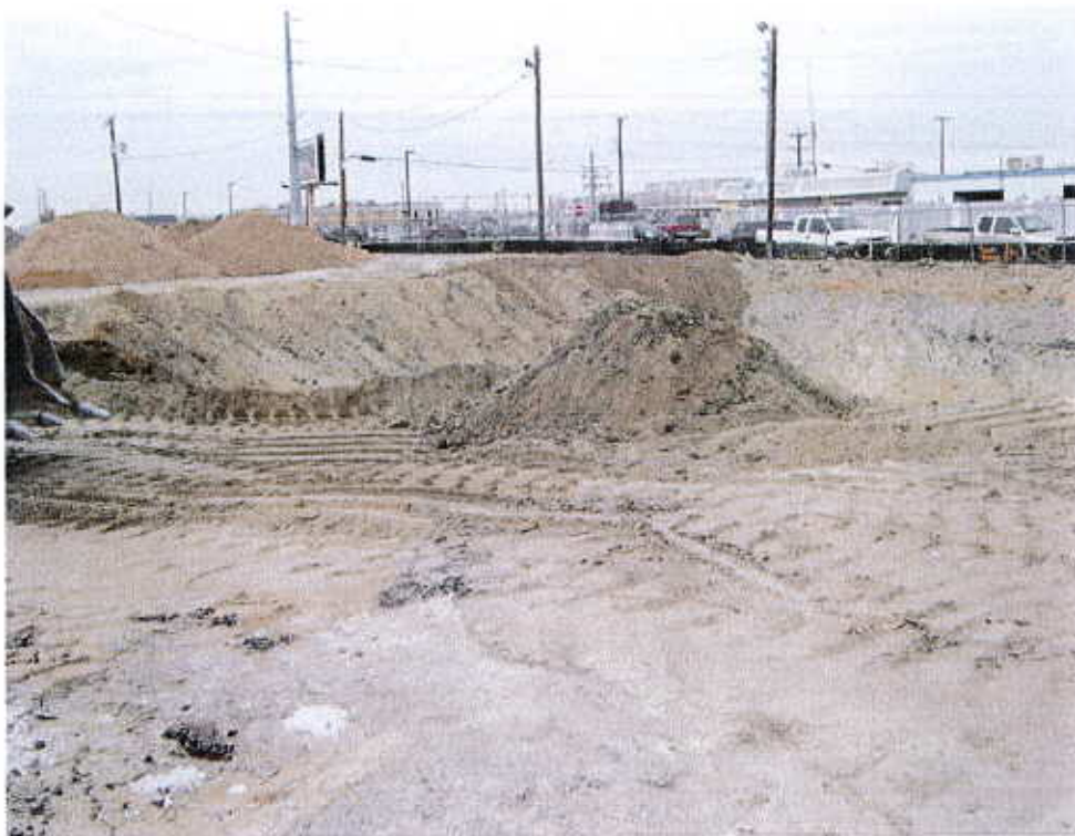
B.3, Segregation of TPH Soil and Clean Backfill, Southeast to Northwest View
