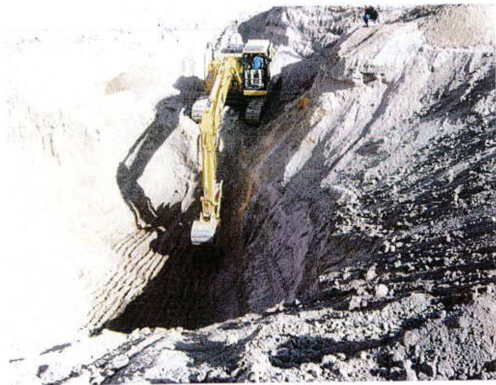
B.11, Obtaining Soil Samples from Bottom of Excavation Cavity
