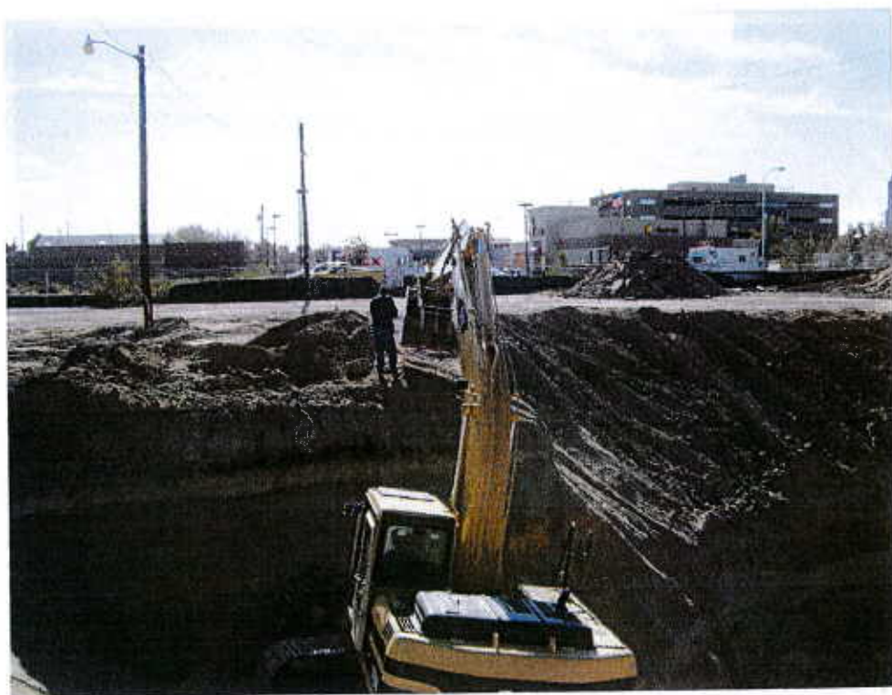
B.12, Obtaining Soil Samples from Bottom of Excavation Cavity
