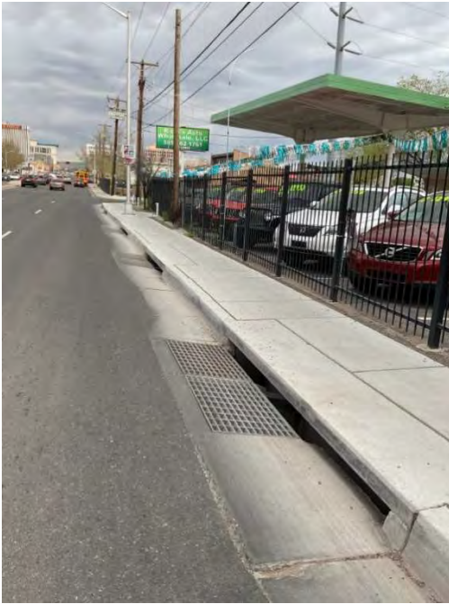
Figure 8: High-Capacity Inlets in Broadway
