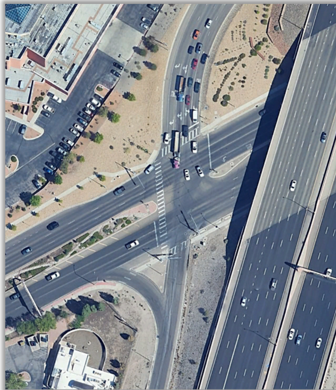
Figure 1 - Lomas Blvd NE and I-25 Southbound On-Off Ramp
