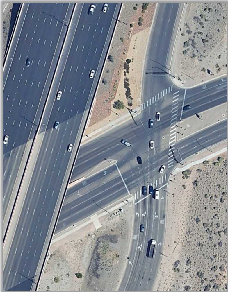
Figure 2 – Lomas Blvd NE and I-25 Northbound On-Off Ramp
