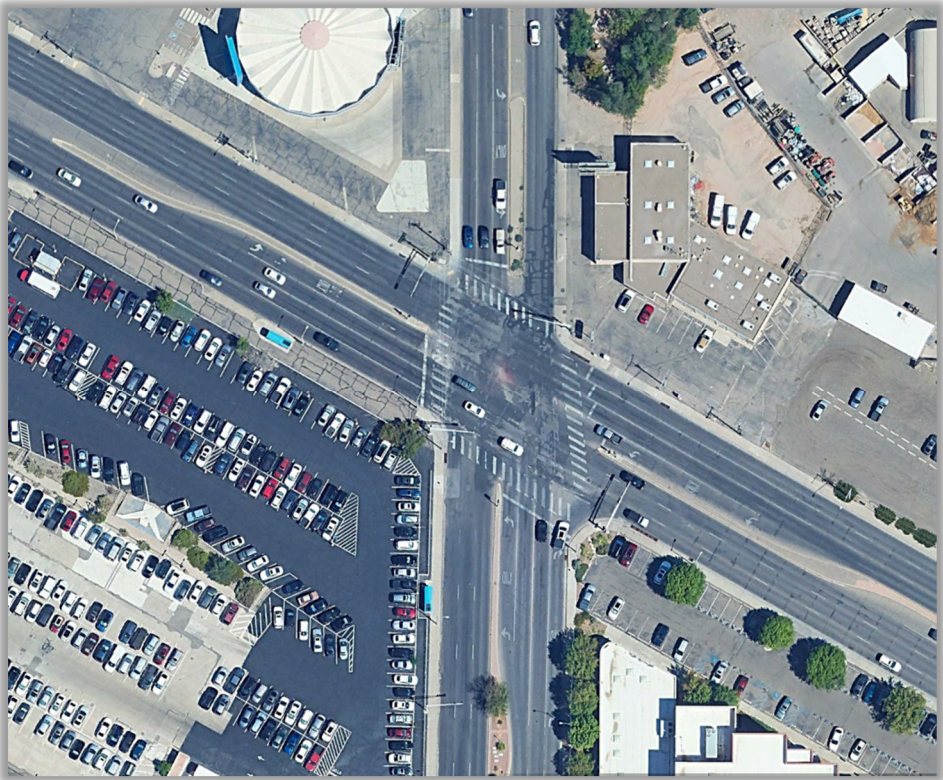
Figure 3 – Lomas Blvd NE and University Blvd NE
