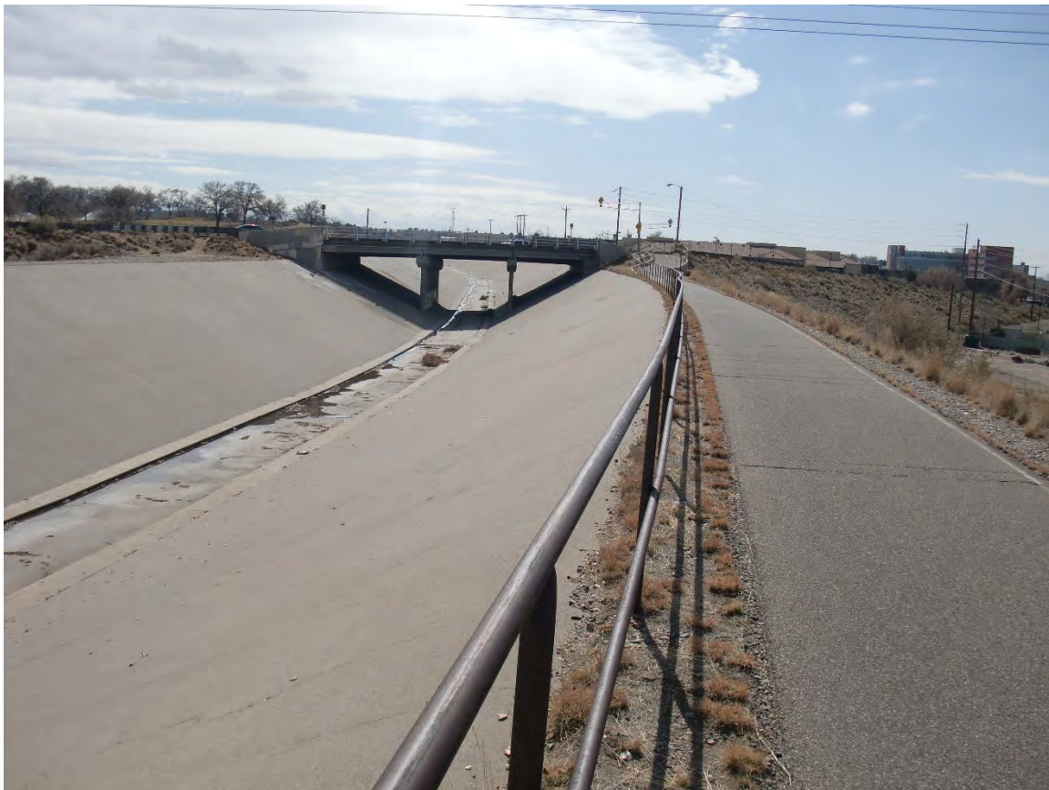
Figure 2 - North Diversion Channel – Looking Upstream (South)
