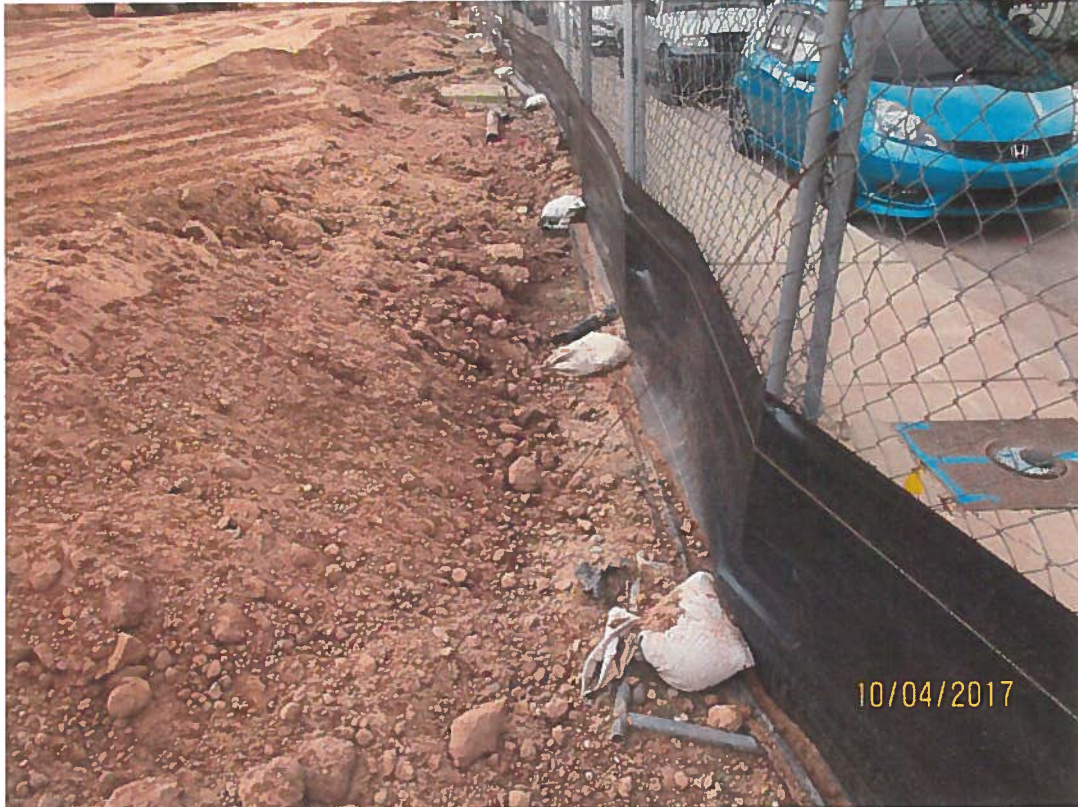
Silt fence not buried/sealed.
