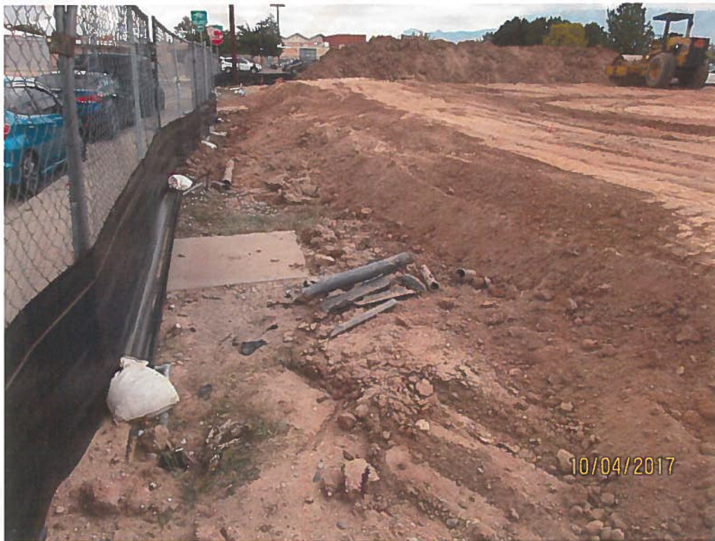
Silt fence not buried/sealed.
