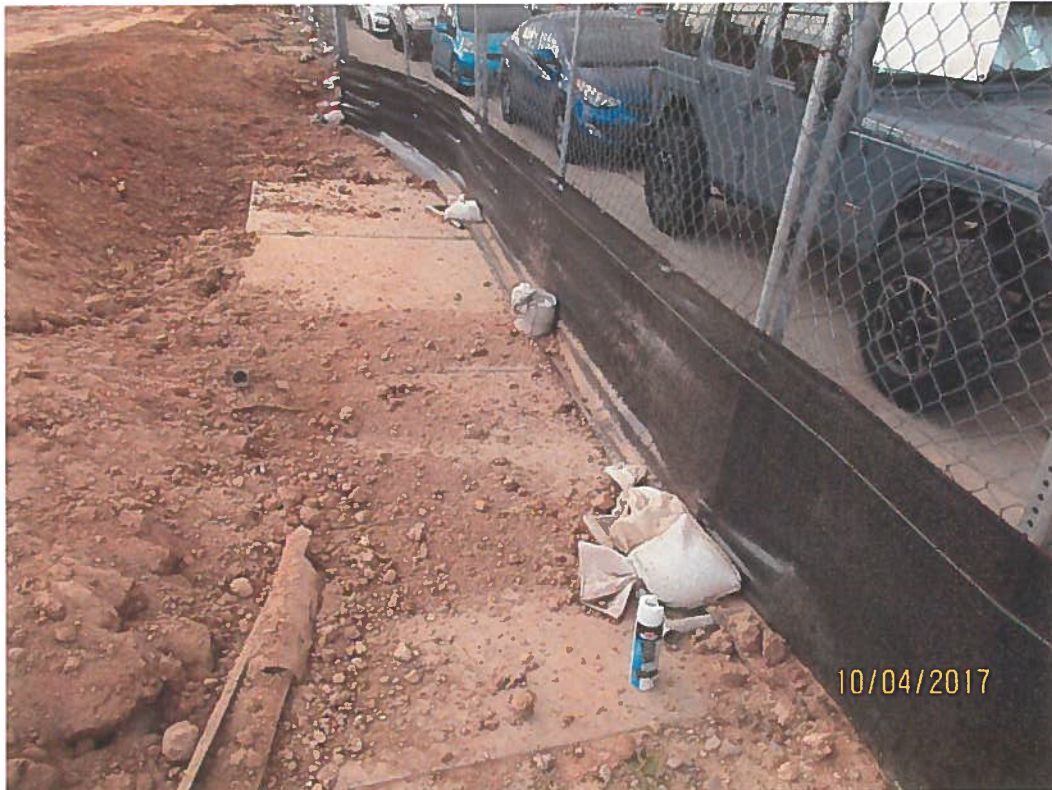
Silt fence not sealed on concrete surface.
