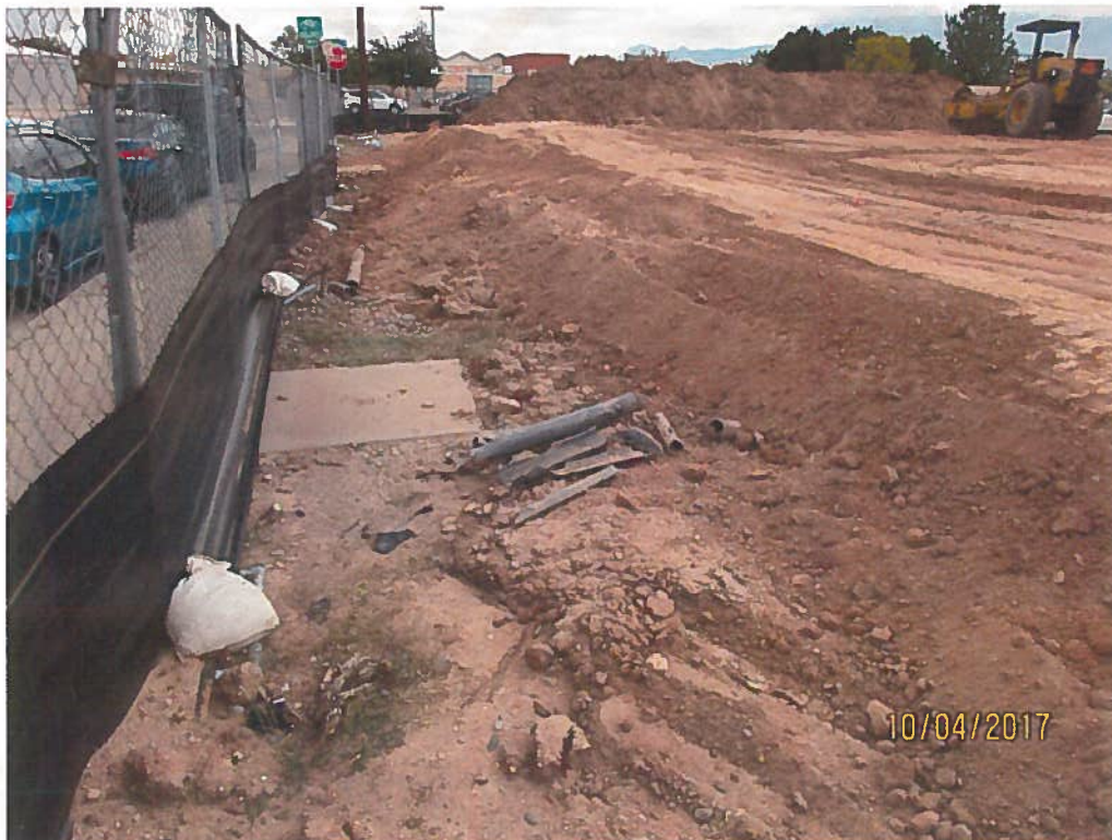
Silt fence not buried/sealed.
