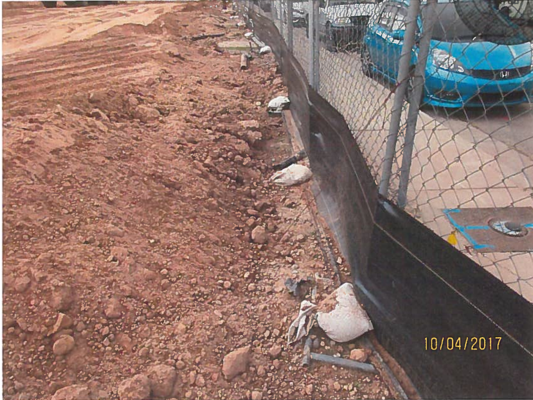
Silt fence not buried/sealed.
