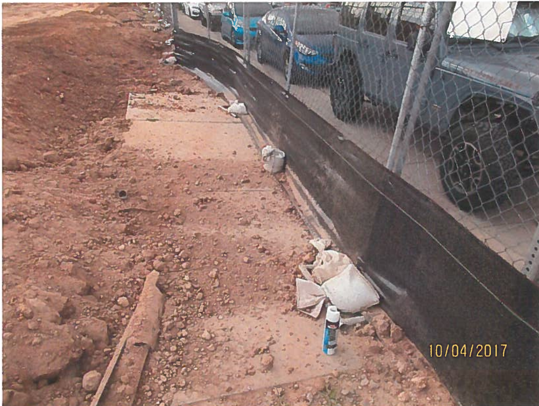
Silt fence not sealed on concrete surface.
